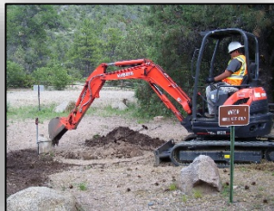
Waterline and hydrant repairs at Cayuse Trailhead
