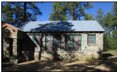
Historic Groom Creek Schoolhouse received roof and window repairs in 2014.
