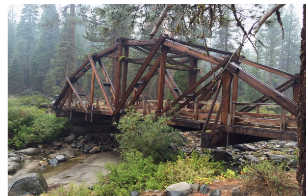
Historic Dinkey Creek Bridge. Built in 1938, it was the first "bowstring arch truss" bridge built in California.
