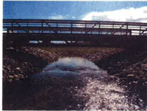
Figure 8-5. Portage Creek Rock Rapids and Bridge
