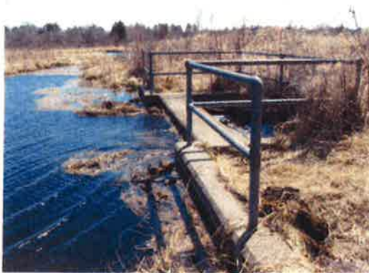
Figure 8-4. Portage Creek Dam
