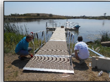
Contractors install a new fishing pier at Sather Lake.
