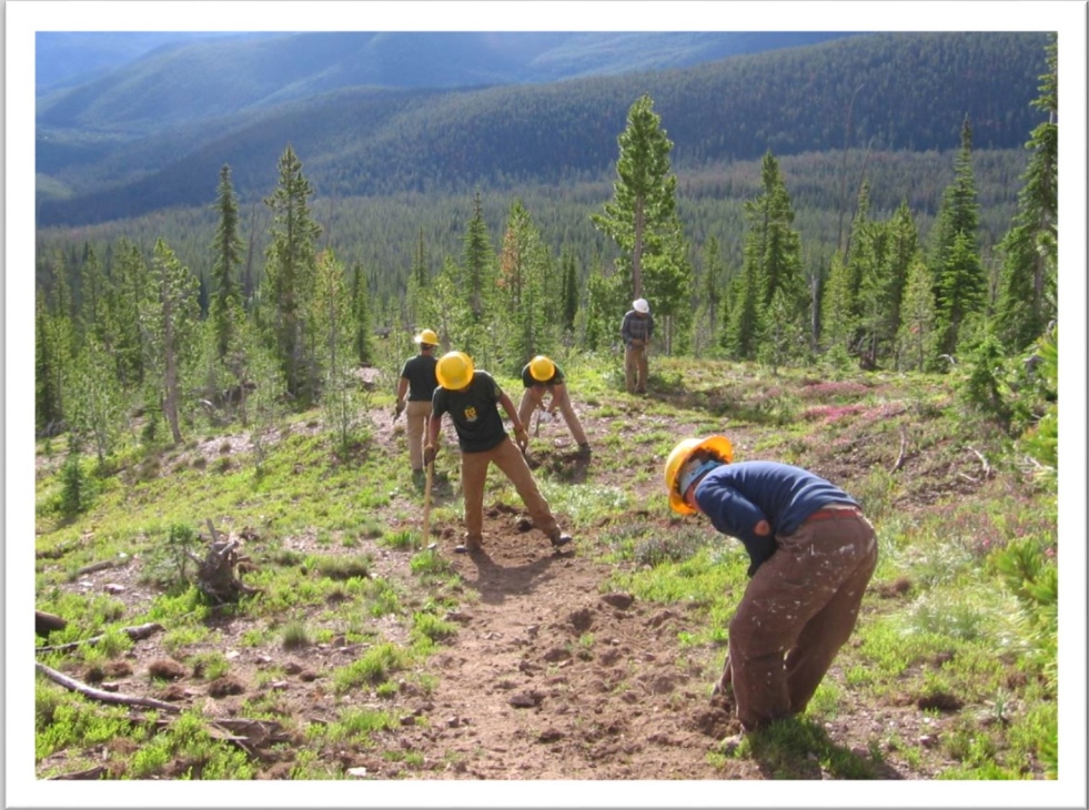
MCC Crew - Dwight Creek Trail Reconstruction
