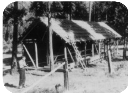
Above: Moose Creek Parachute Loft, Earl Cooley photograph
