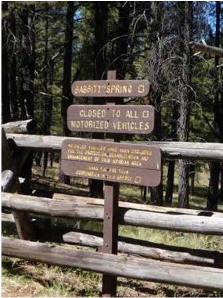
Figure 14. New Babbitt Spring information signs installed on the rebuilt log pole fence.
