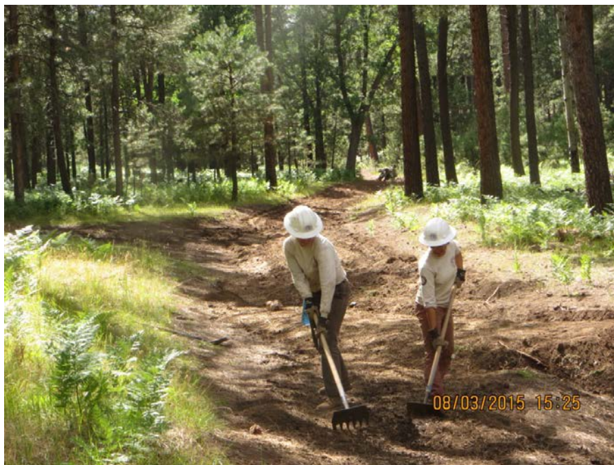
Figure 4. Recontouring and re-seeding of a non-system road to restore forest vegetation by American Conservation Experience (ACE)
