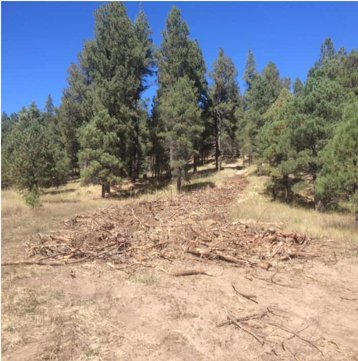
Figure 9. Soft closure of non-system road off of Forest Road 762 using logging slash
