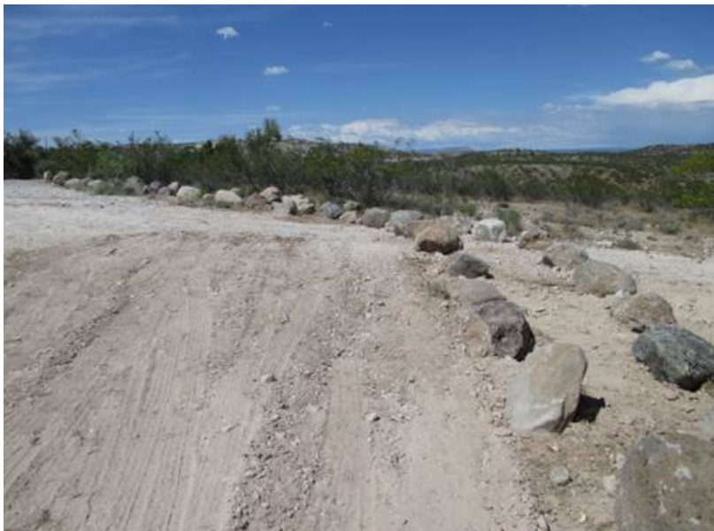
Figure 8. A double-wall of boulders to reduce unauthorized motor vehicle use
