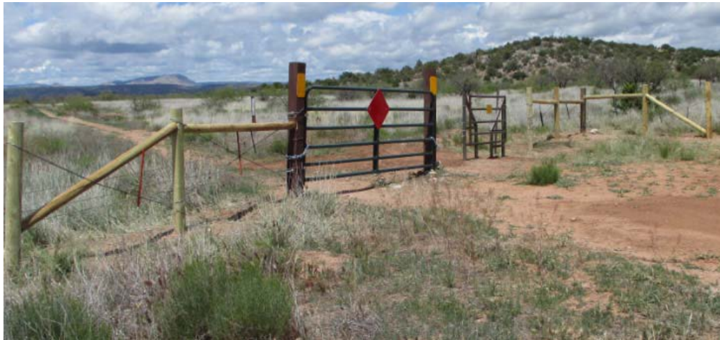
Figure 13. Gate and fencing installed on 9203C to reduce unauthorized motor vehicle use
