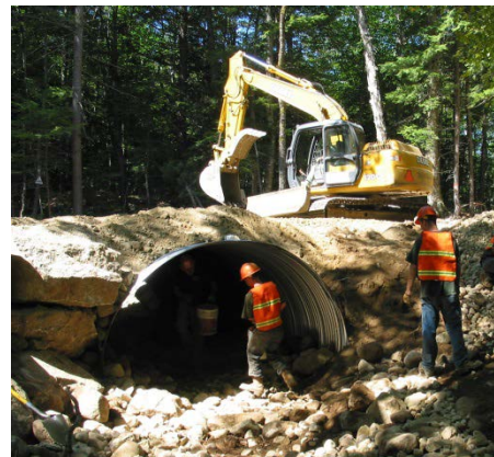
Culvert replacement to improve fish passage. WMNF photo.
