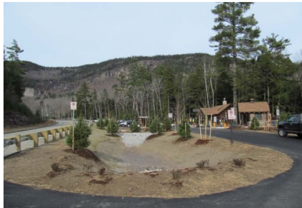
Lower Falls Day Use Area after reconstruction. WMNF photo by Sheela
