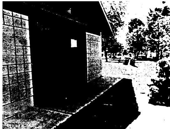
Figure 9. --In modern settings, well-developed toilet facilities may be provided for convenience of visitors; in more rustic settings, they may be for safety of visitors or for protection of resources.
