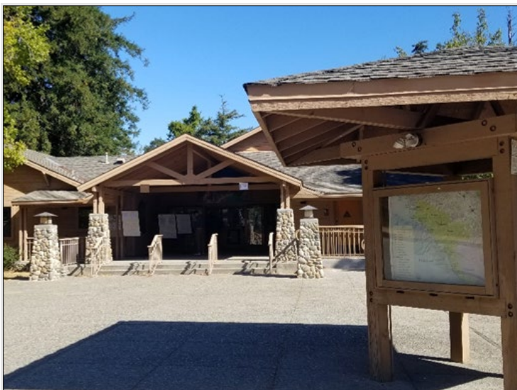
Figure 12. Multi-Agency Facility, Big Sur Station
