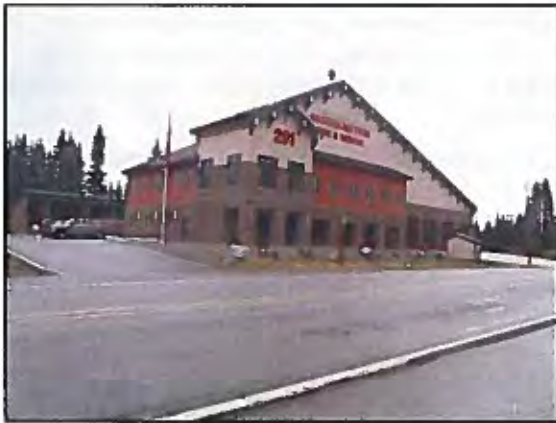
New trailhead and parking near Snoqualmie Pass Fire Station for PCT south access
