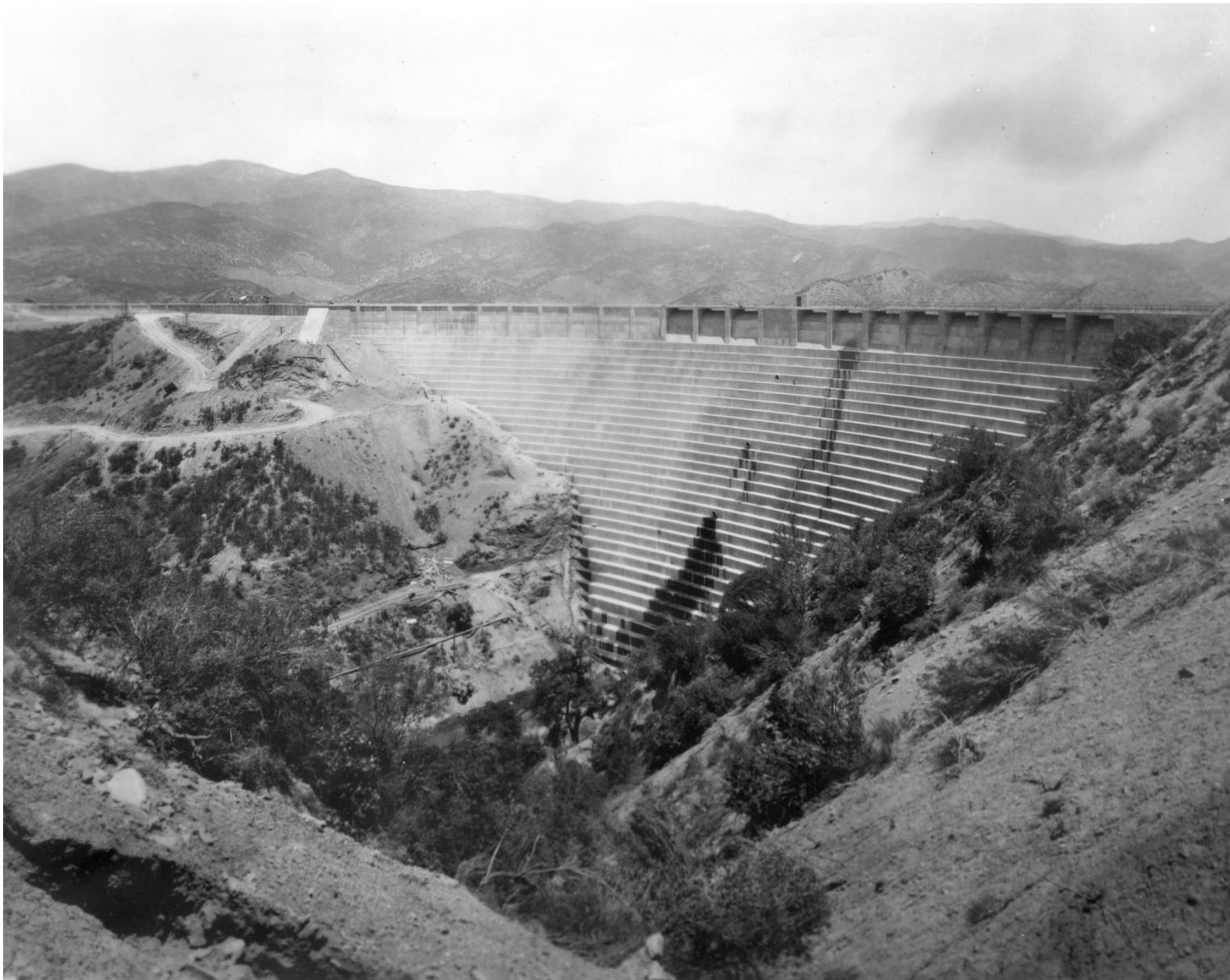
Saint Francis Dam in San Francisquito Canyon near Saugus, CA, before it failed in 1928. This pre-failure photograph shows the exterior of the dam and surrounding countryside. Some water stains can be seen on the wall. (Photo credit: Security Pacific National Bank Collection/ Los Angeles Public Library)
