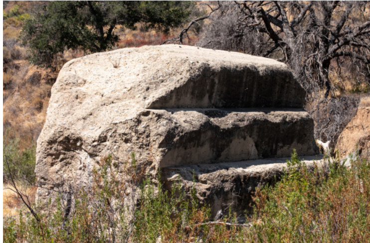
"Block 19", one of the largest remaining parts of the dam
