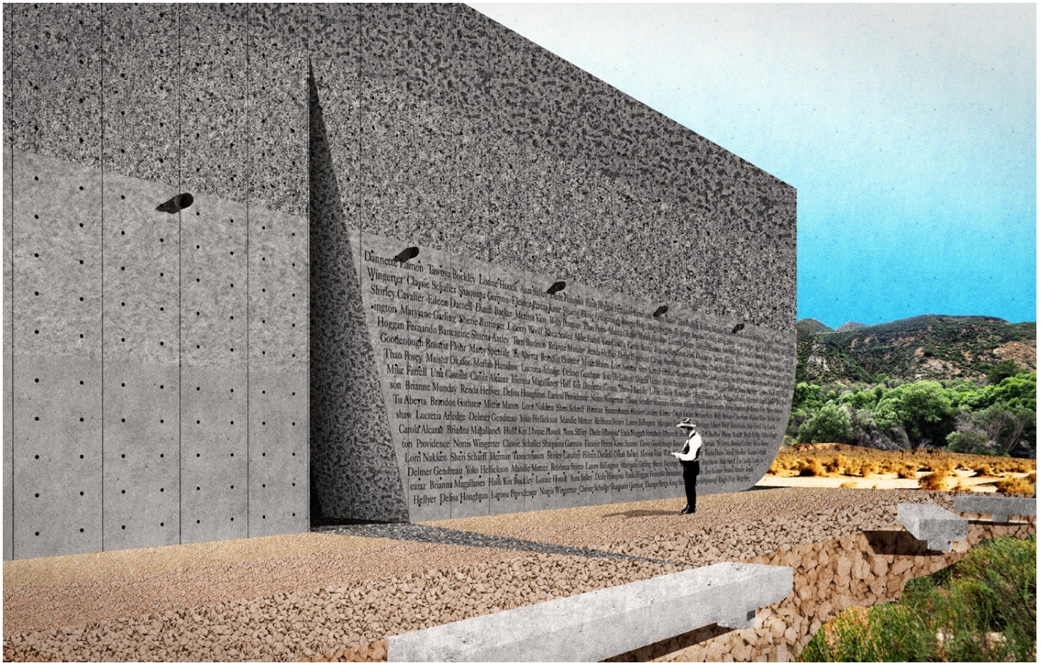
Victims names carved into the concrete face.
