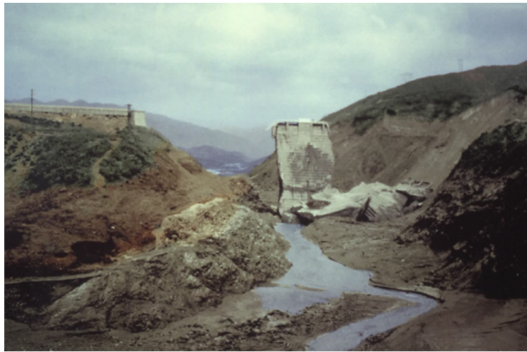
The "tombstone", a section of the dam that remained standing after the disaster and was later demolished.
