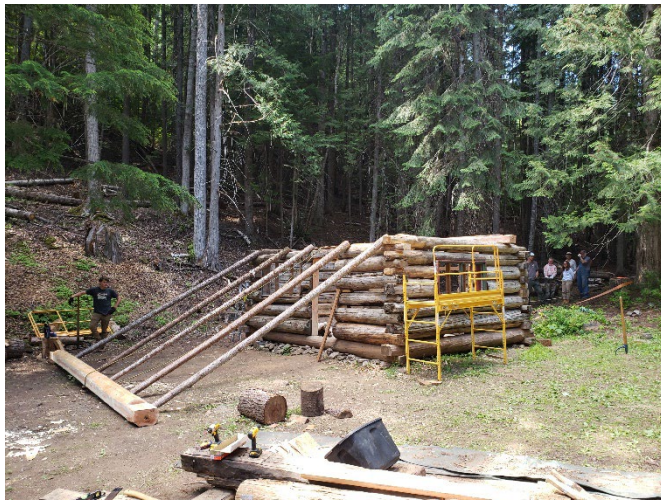
Photo 3: 2023 Raising a log into position at Gypsy Copper Cabin.
