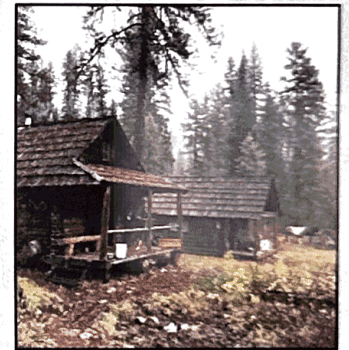
Figure 4: Shearer Guard Station.
