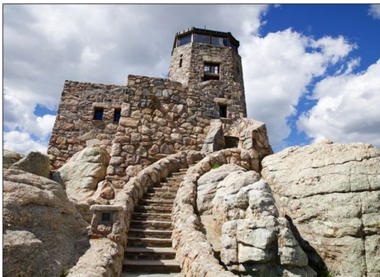
Harney Lookout Tower, on top of Black Elk Peak in the Black Hills National Forest, constructed by the Civilian Conservation Corps during 1935-1938. This is the highest fire lookout in the Black Hills at 7,244 feet. Photo credit - Tripadvisor.com
