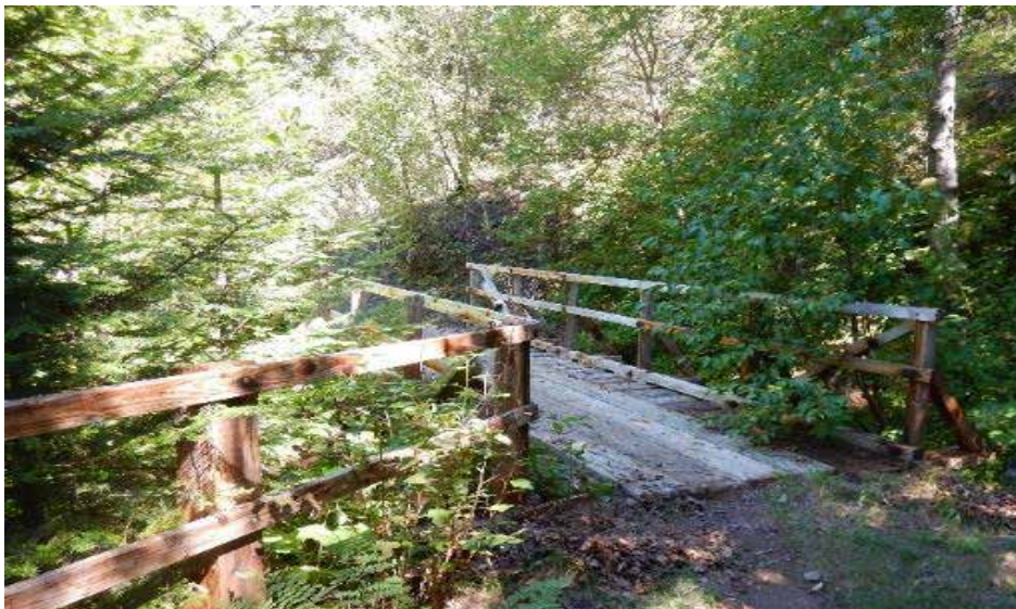
Figure 66. Trail bridge along Fish Creek trail
