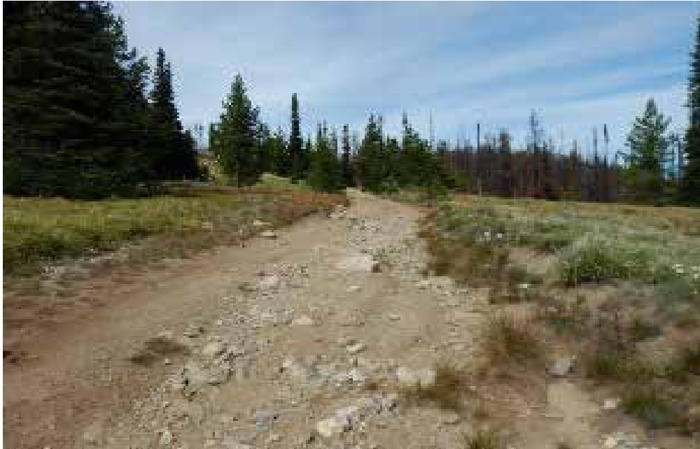
Figure 100. FR466 enters the roadless area from the north
