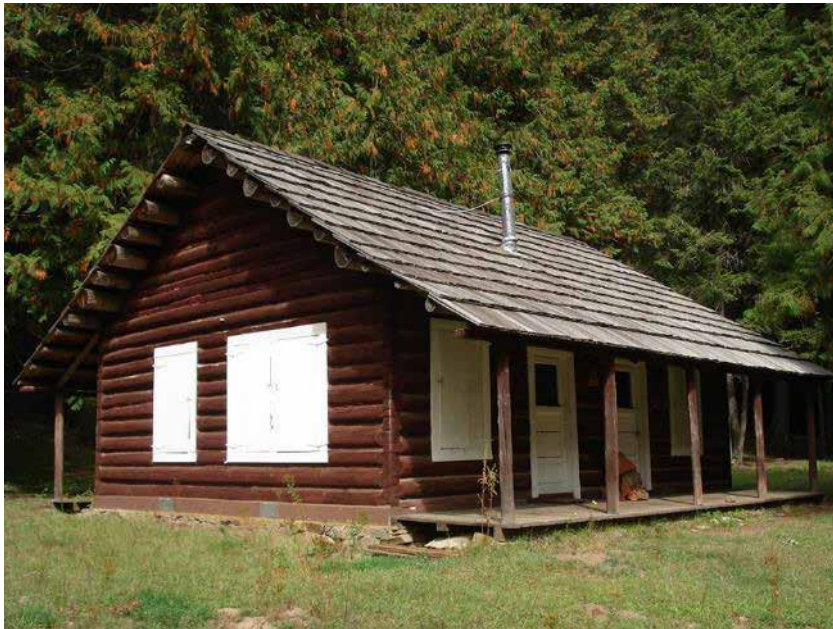
Figure 14. Meadow Creek Ranger Station; now a recreation rental
