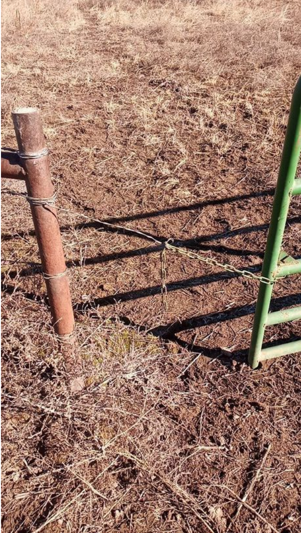
Inadequate gate closure
