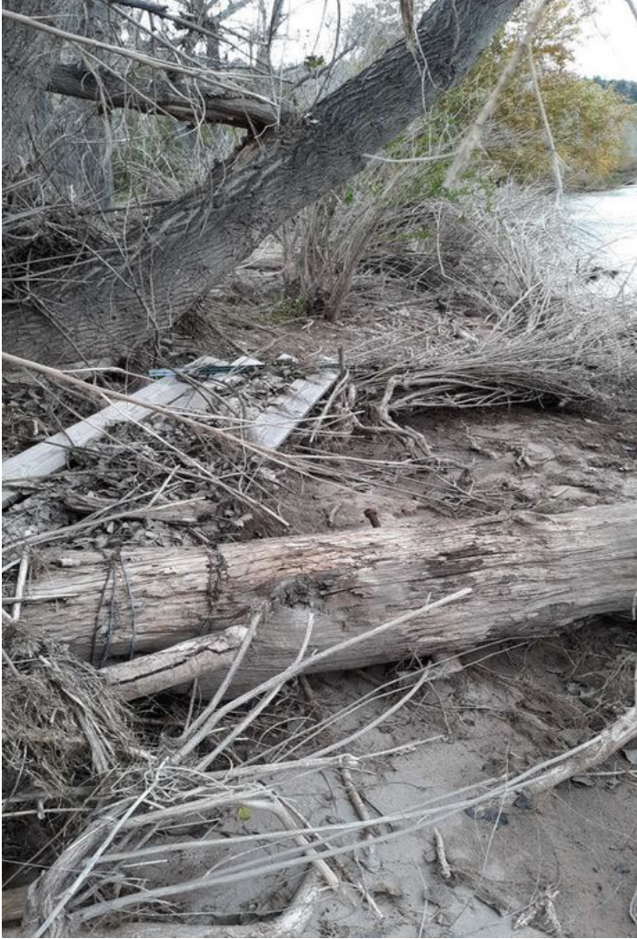
Downed boundary fence at river.
