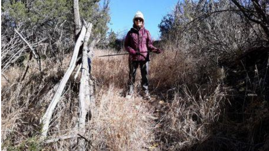
Downed fence east side of river near bridge.
