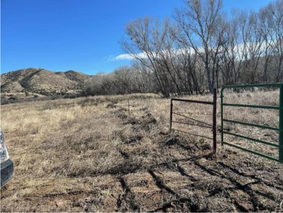
Fence and gate repaired
