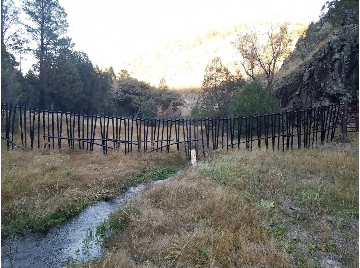
Figure 1. One-way gate at downstream end of enclosure where Beaver Creek exits the enclosure.
