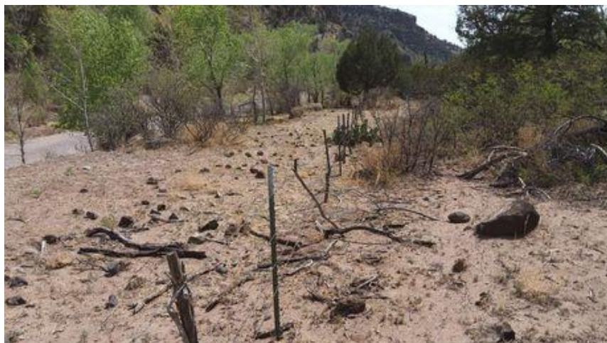
Exclosure fence. Good condition.
