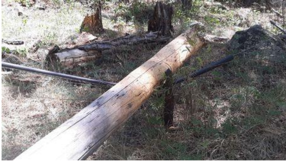
Fence damaged by fallen tree along east side enclosure.
