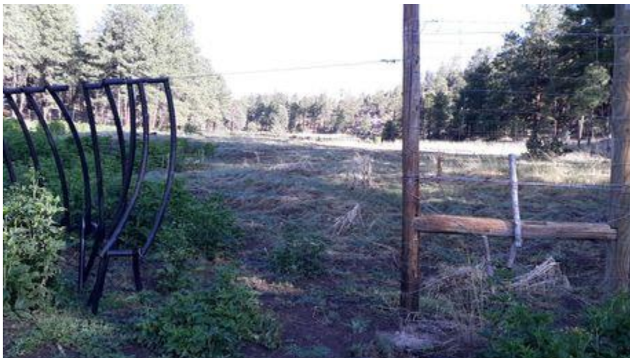
Enclosure piping gap along first elk enclosure.
