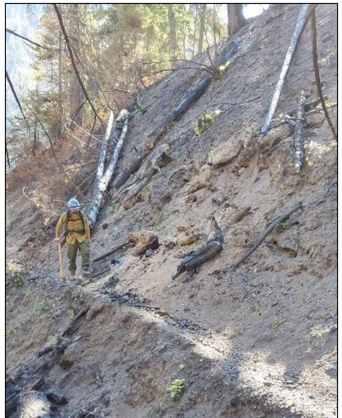
Figure 5 Cedar Creek Trail damage may get worse with eroding hillslopes.
