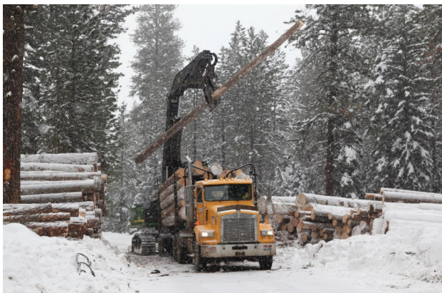
The Southwest Idaho Wildfire Crisis Landscape project will utilize both commercial and non-commercial timber harvesting. Waiting until the ground is frozen helps in erosion control and soil disturbance. Photo courtesy of the Payette National Forest
