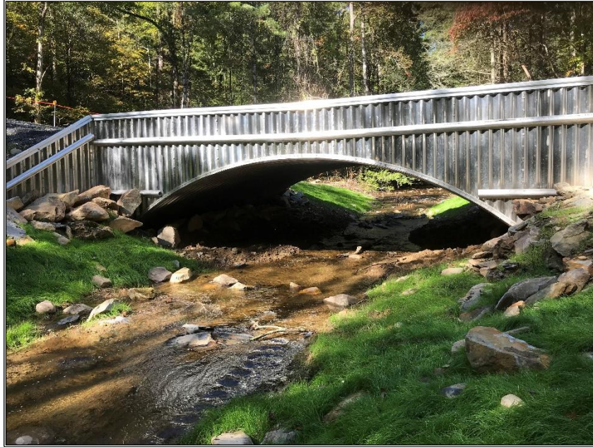
A new bottomless culvert is on Mill Creek near the beginning of the Rocky Flats OHV trail.
