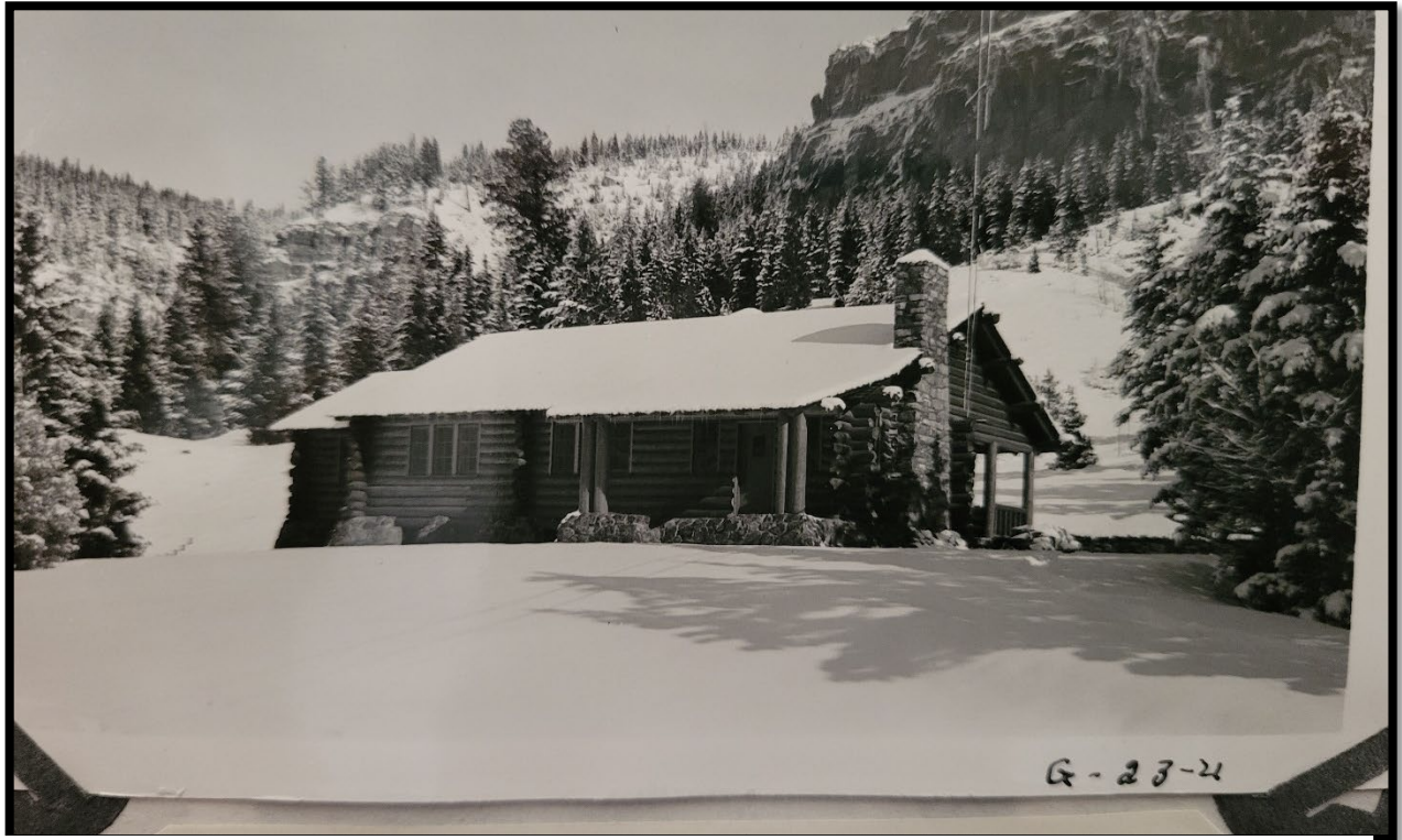
Figure 17. Ranger's residence newly completed circa 1936
