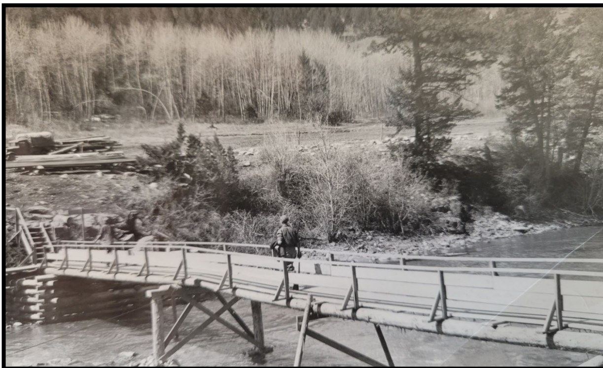
Figure 13. Temporary footbridge over Gallatin River for bridge construction April 26, 1935
