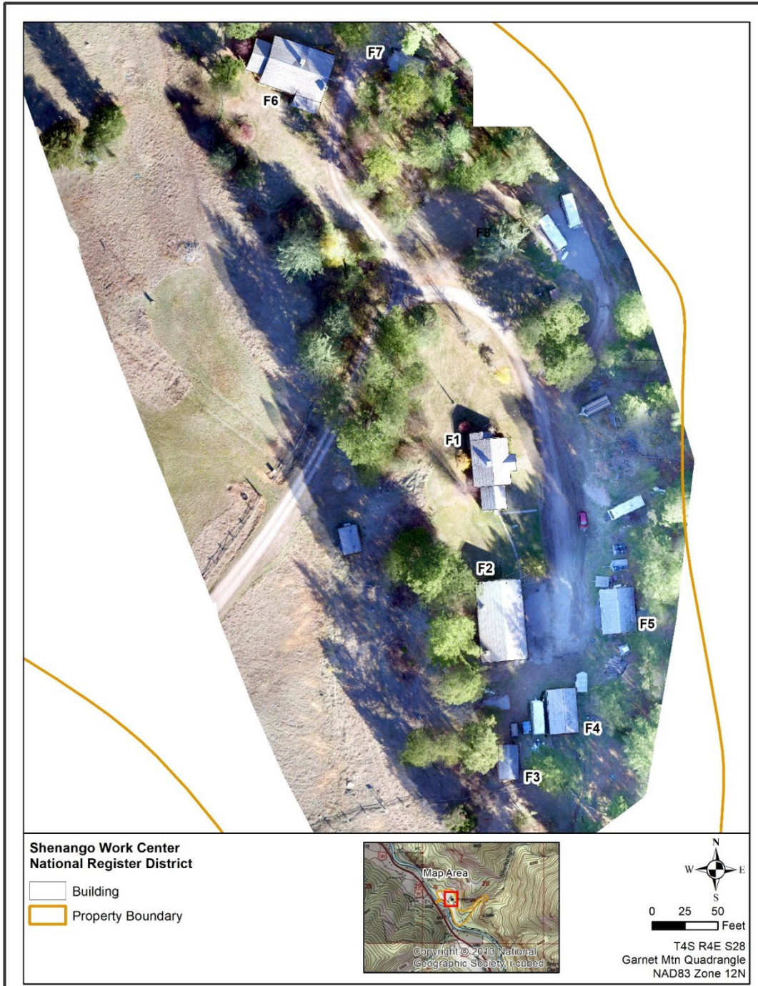
Sketch map with UAV derived orthoimage showing detailed layout of concentration of CCC era buildings on property
