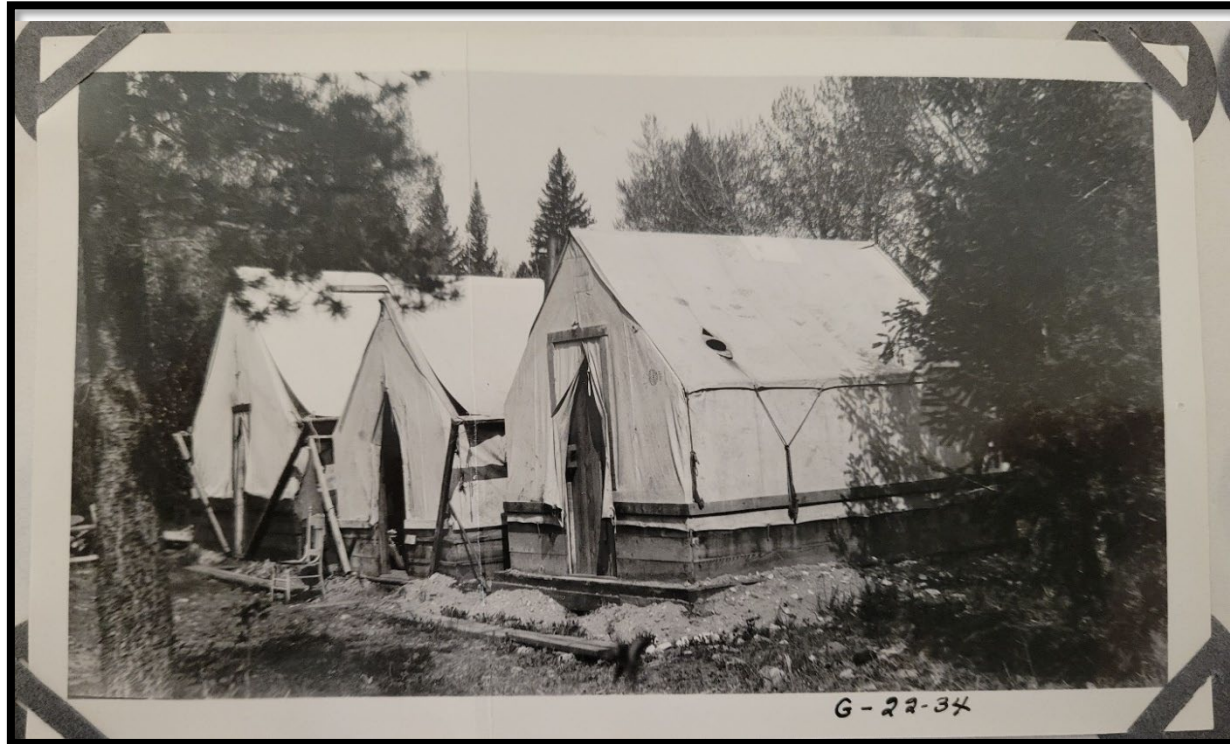
Figure 3. Example of temporary tent camps at Squaw Creek CCC camp in 1934
