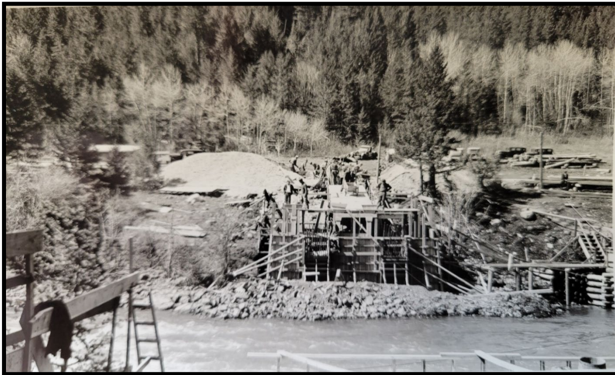
Figure 14. Bridge forms beginning to be put in place 1935
