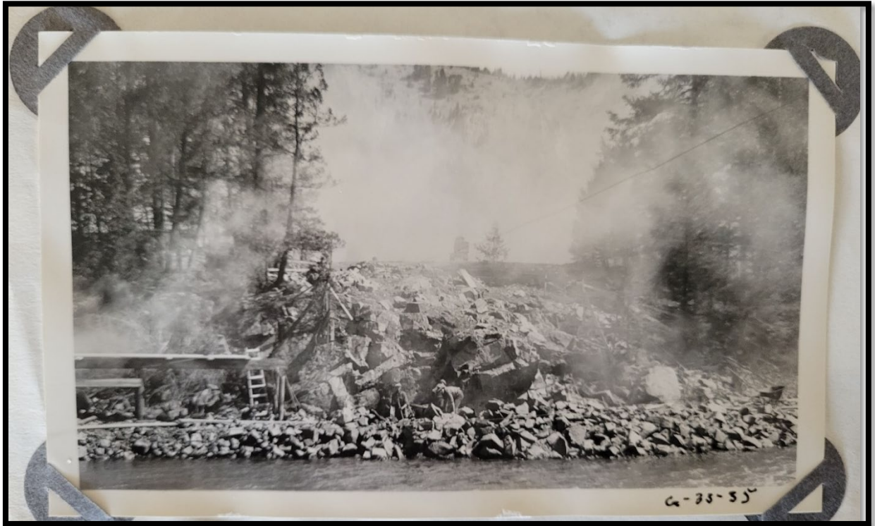
Figure 11. View of excavation for concrete footings with dynamite looking at east side of river April 26, 1935
