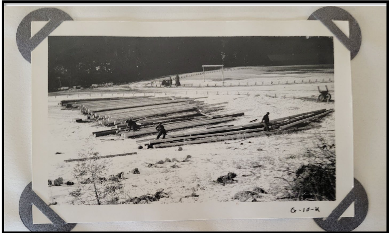
Figure 9. Men peeling logs for new ranger station December 20, 1935
