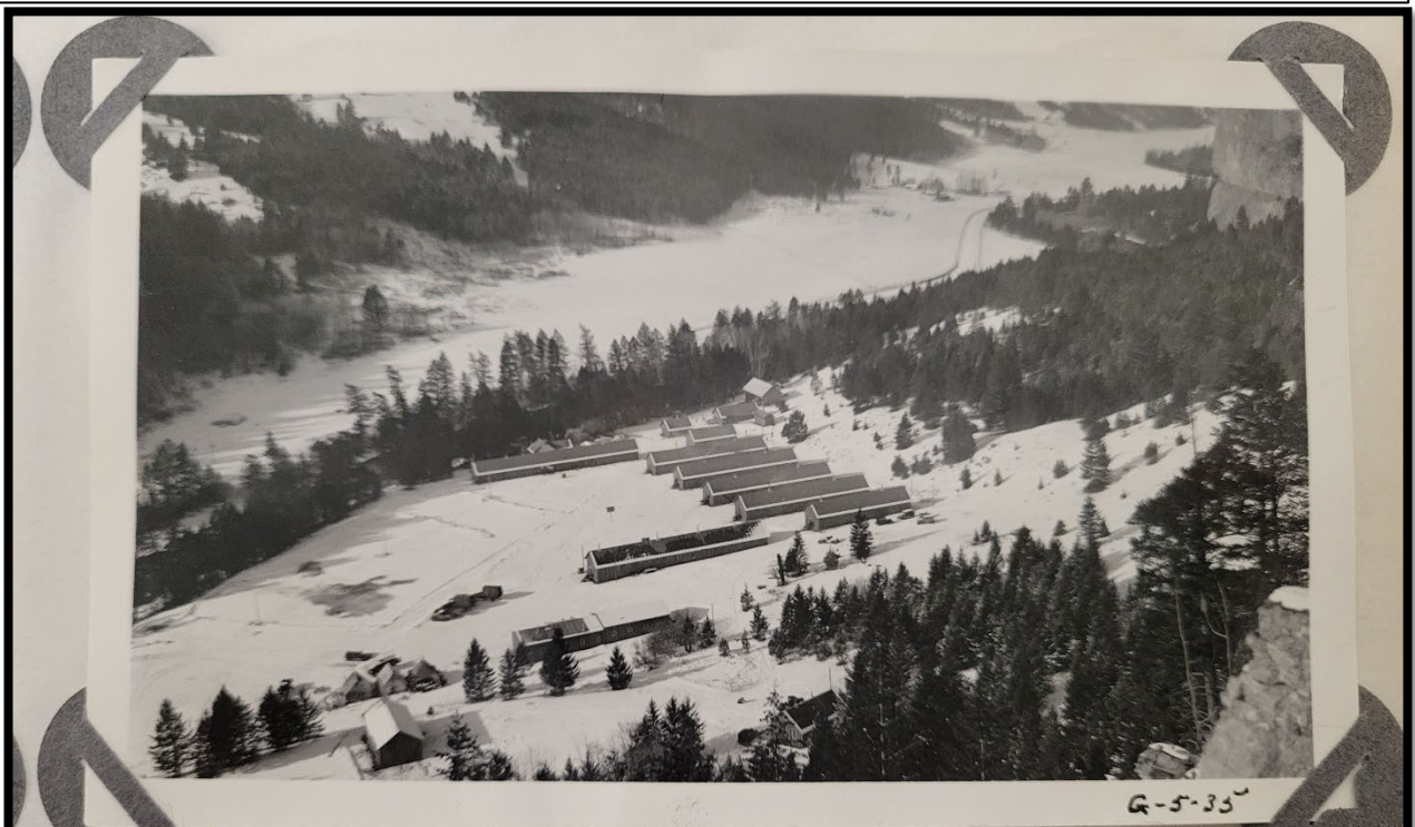
Figure 10. Completed CCC camp D-F-57 overview as of January 9, 1935
