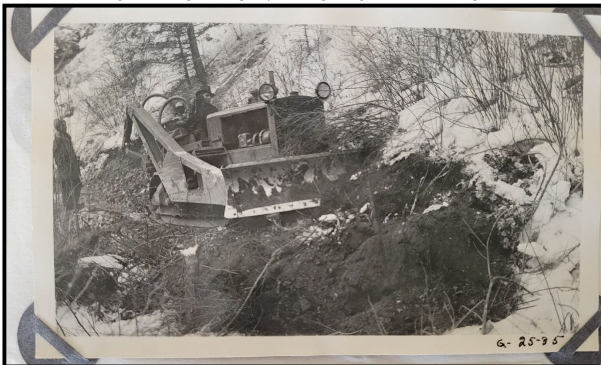
Figure 4. Road building activities from January 9, 1935
