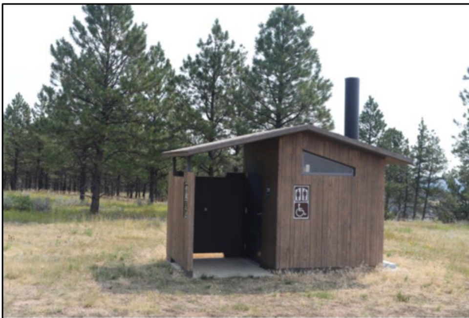
MT_RosebudCounty_PokerJimButteLookout_0007. Looking East at the (noncontributing) latrine, Site 24RB2233, Poker Jim Butte Fire Lookout August 26, 2021, View to East (Urbaniak 2021)
