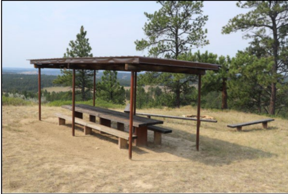
MT_RosebudCounty_PokerJimButteLookout_0008. Looking Southwest at the (noncontributing) picnic shelter and associated benches, Site 24RB2233, Poker Jim Butte Fire Lookout August 26, 2021, View to Southwest (Urbaniak 2021)
