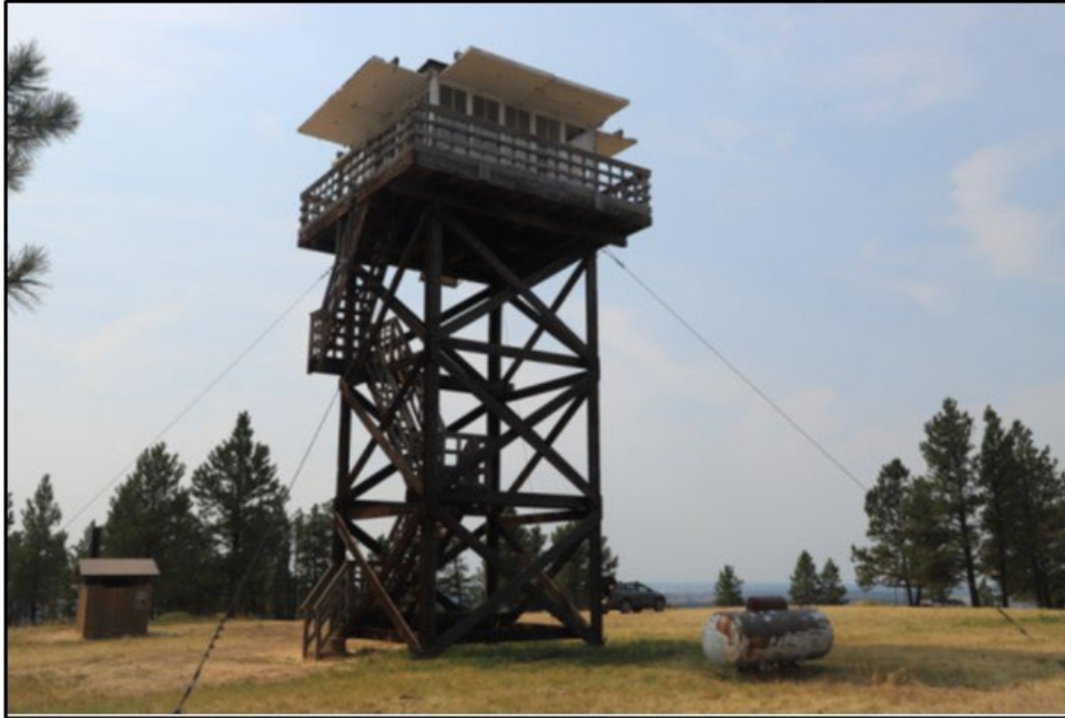
MT_RosebudCounty_PokerJimButteLookout_0006. Looking Southwest from the Northeast side of the tower showing proximity of propane tank and latrine, Site 24RB2233, Poker Jim Butte Fire Lookout August 26, 2021, View to Southwest (Urbaniak 2021)
