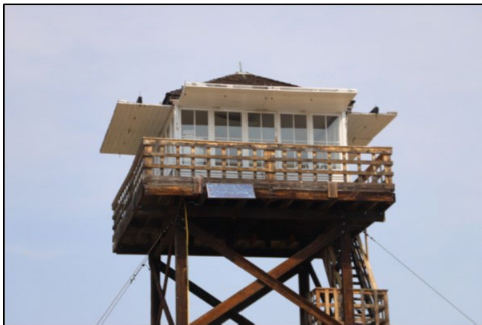
MT_RosebudCounty_PokerJimButteLookout_0003. Lookout Cabin, Site 24RB2233, Poker Jim Butte Fire Lookout August 26, 2021, View to North (Urbaniak 2021)
