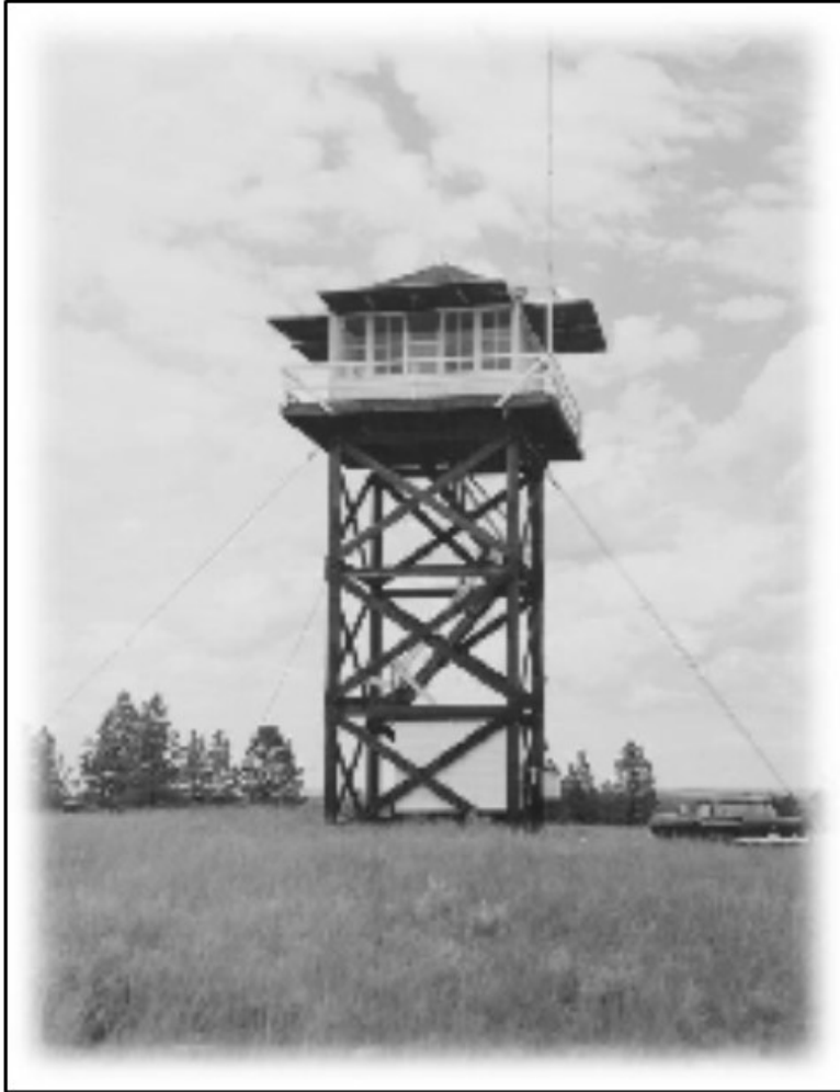
MT_RosebudCounty_PokerJimButteLookout_0013. The Poker Jim Butte Fire Lookout in 1962 with storage area present in bottom southwest corner of tower, Site 24RB2233, Poker Jim Butte Fire Lookout
