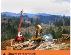
▲ Shovel yarder truck
