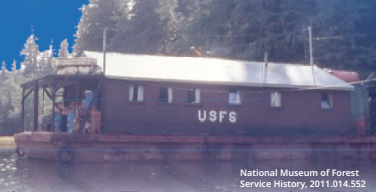
A wanigan (often spelled wannegan) is a temporary shelter towed by boat or truck. The Forest Service towed this wanigan to Kuiu Island in Tongass National Forest in 1971 to serve as crew living quarters.
