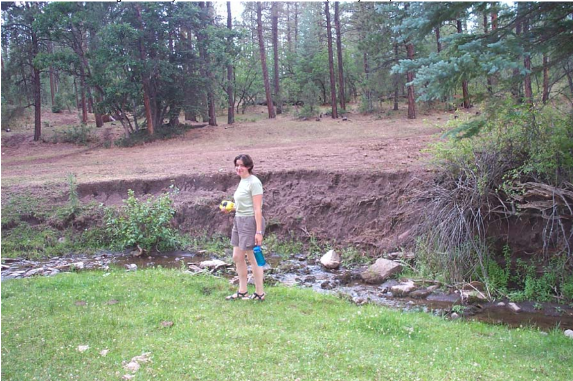
Photo 48. Bank instability on Capulin Creek caused by heavy grazing and recreation on a spur of FS Road 1161 (17 July 2002).
