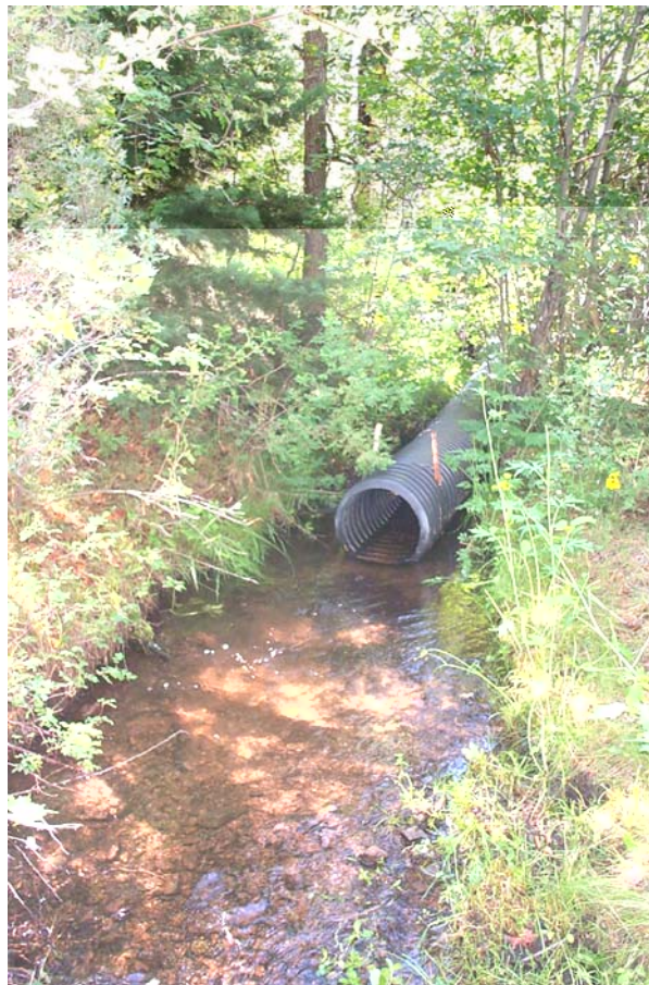
Photo 31. Rito de los Pinos is 100% diverted into this ditch,
