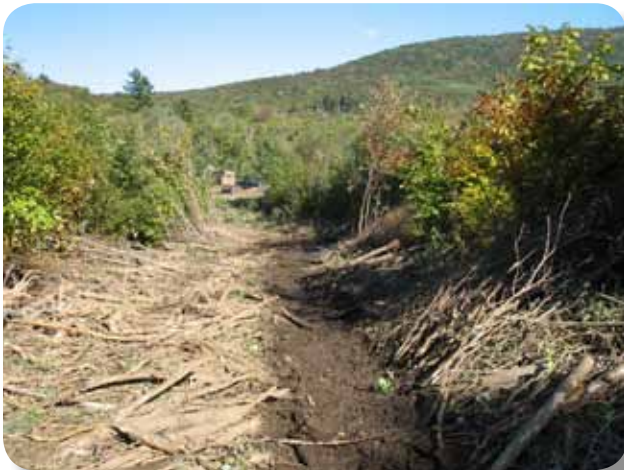
Figure 8. Main skid trail at the Hillock sale on the Pemigewasset Ranger District. The photo was taken in the fall, and looks towards the landing. Slash is layered according to BMPs to minimize rutting and compaction impacts. WMNF Photo by Andy Colter.
