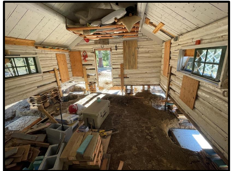
Interior of cabin during jacking process showing new concrete footers poured.
