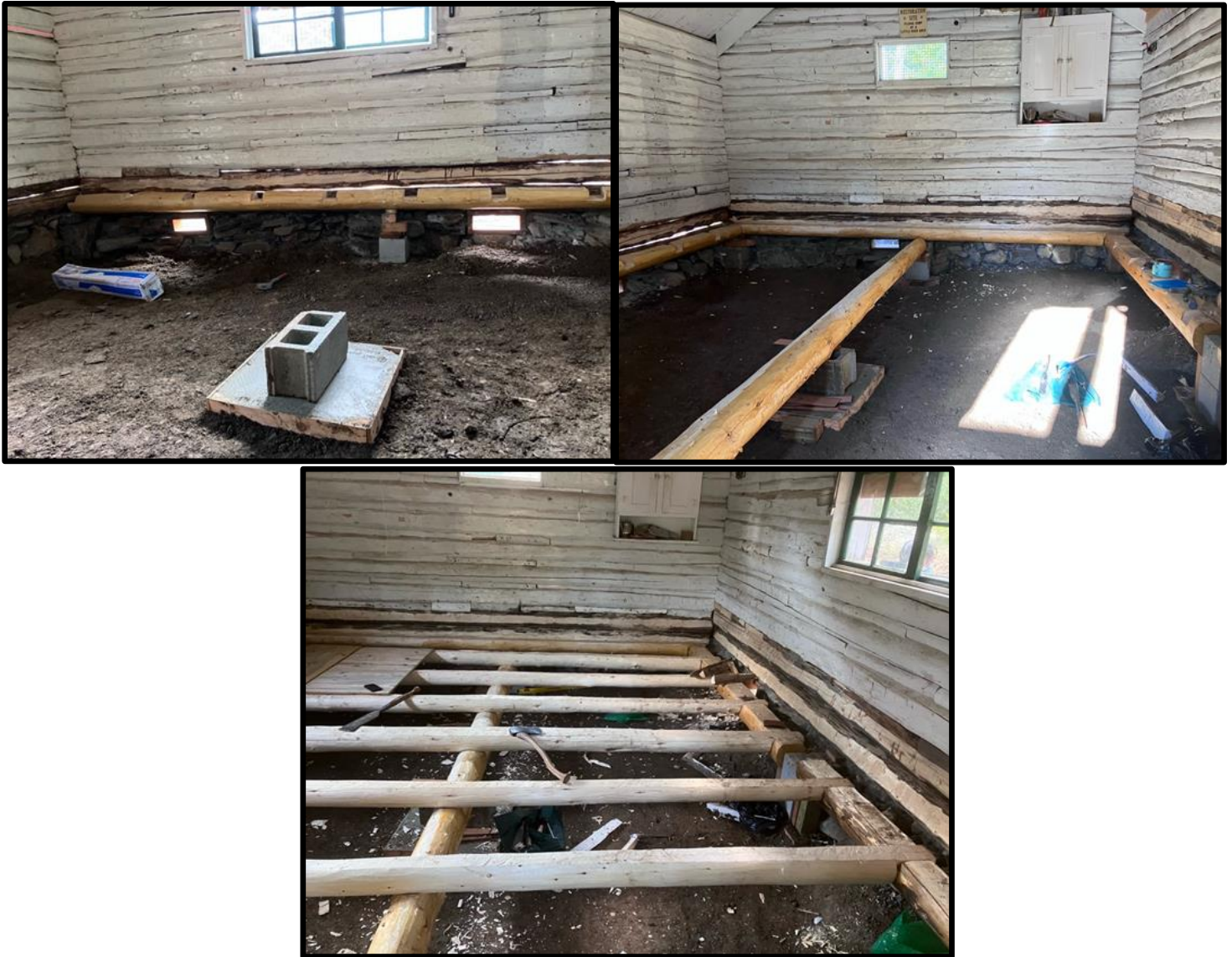
Floor joist construction.
