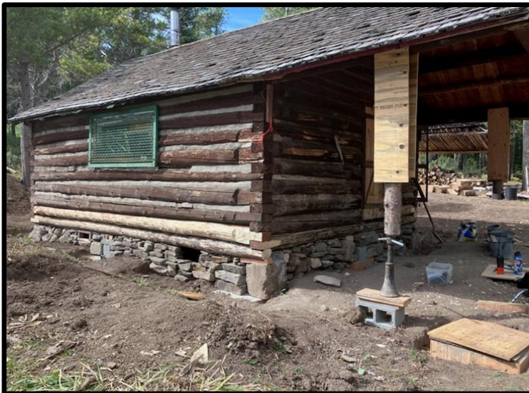
All sill and spandrel logs replaced and rock work begins.
