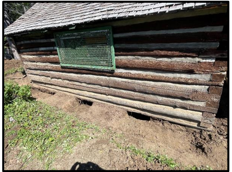
Holes for concrete footers and jacking locations are partially excavated.
