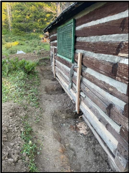
Whalers for jacking the cabin are installed.
