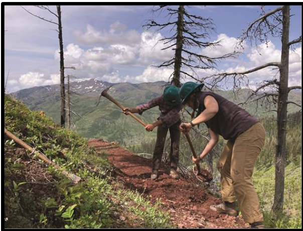
Two interns with BMWF's 2024 Wilderness Conservation Crew improving tread up Falls Point
