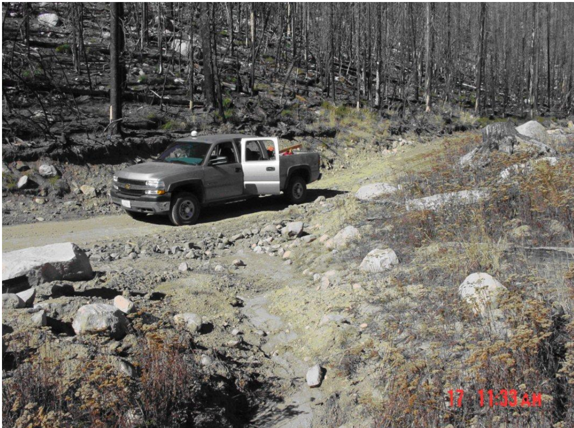
Photo J. A broad based dip with a vehicle parked at the midpoint.
