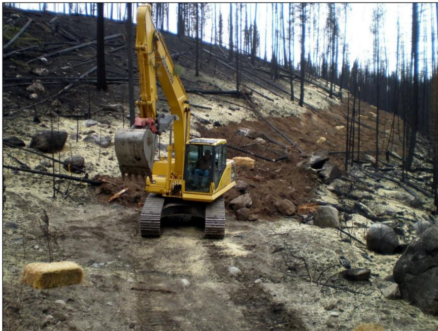
Photo A. Recontoured road.
