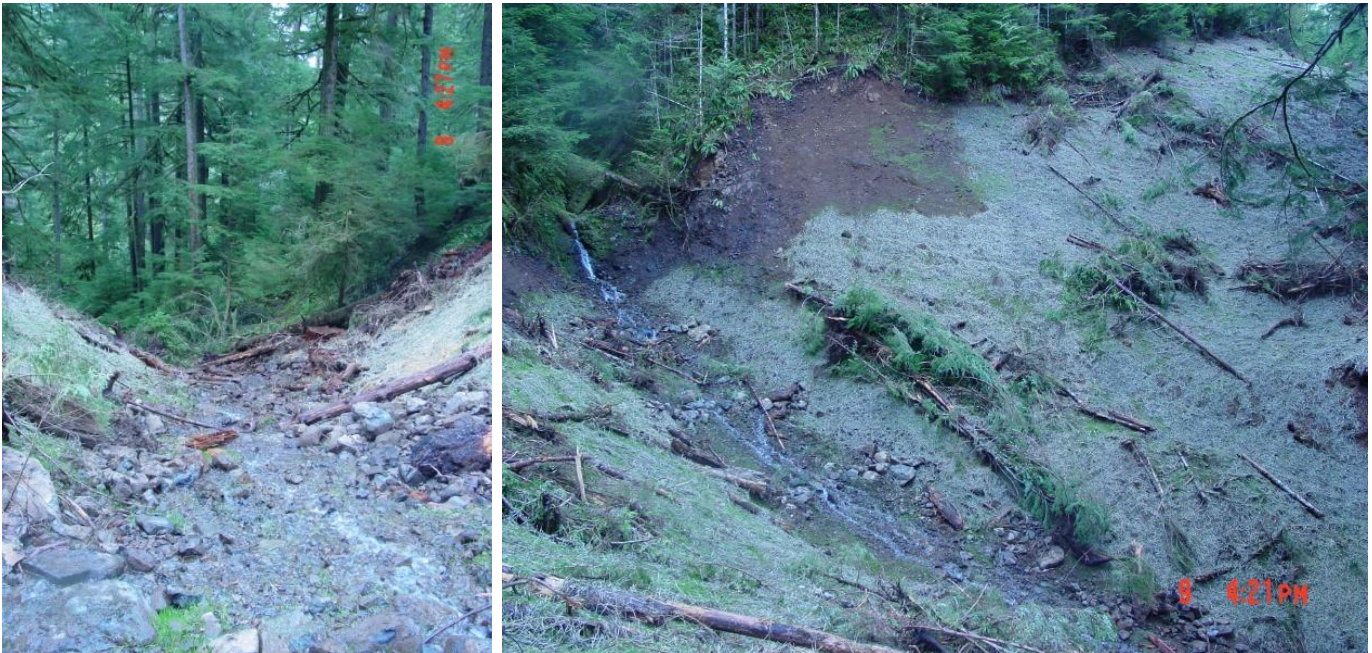
Photo N. Two views of an excavated stream crossing. Notice the straw and logs on the side slopes.
