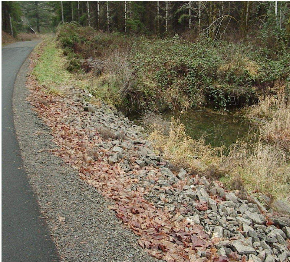
Photo U. A Constructed sump in good condition.
