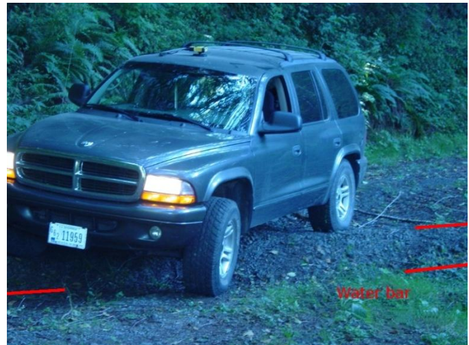
Photo W. Another annotated water bar, with the top and bottom of the water bar marked.
