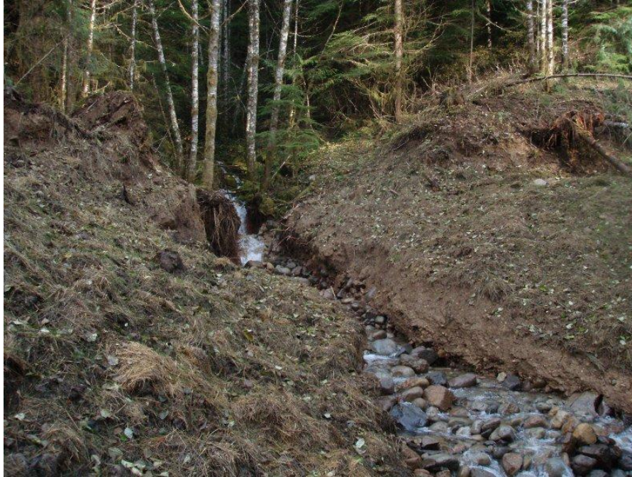
Photo O. This excavated stream crossing has been incised.
