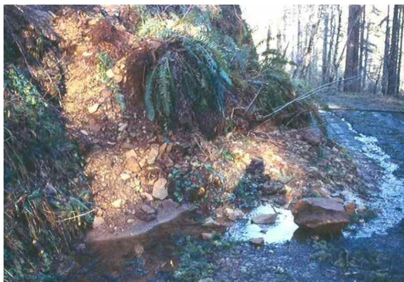
Photo DD. This road related landslide resulted from an over steepened cutslope that failed during an intense rainfall event.
