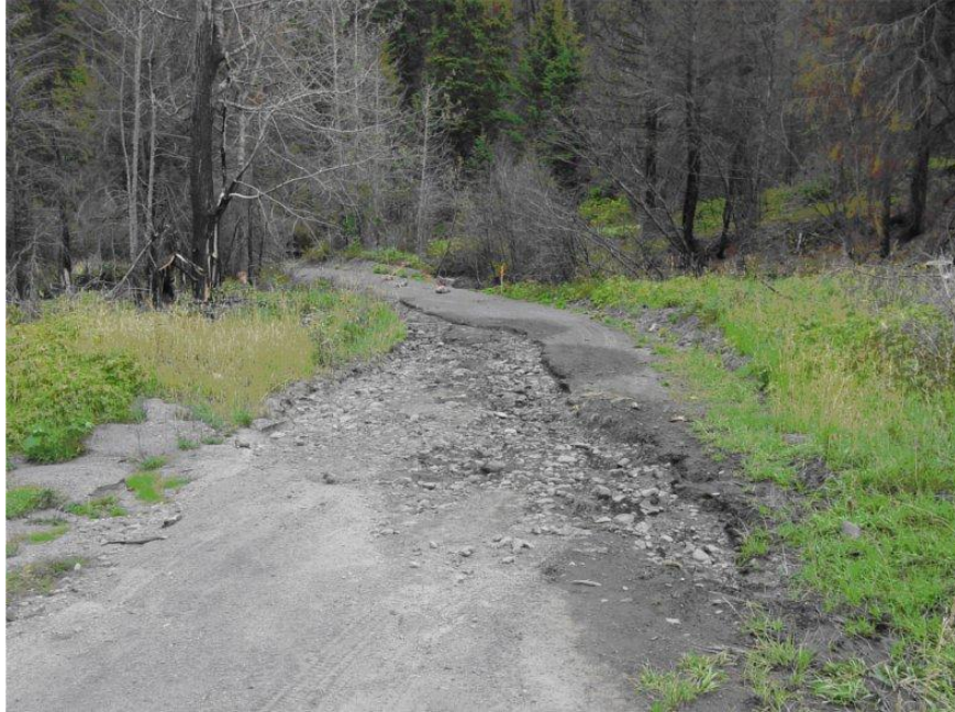
Photo M. Scour of the road surface resulting from capture of an ephemeral channel by the road. Flow Diversion is Yes at this drain point.
