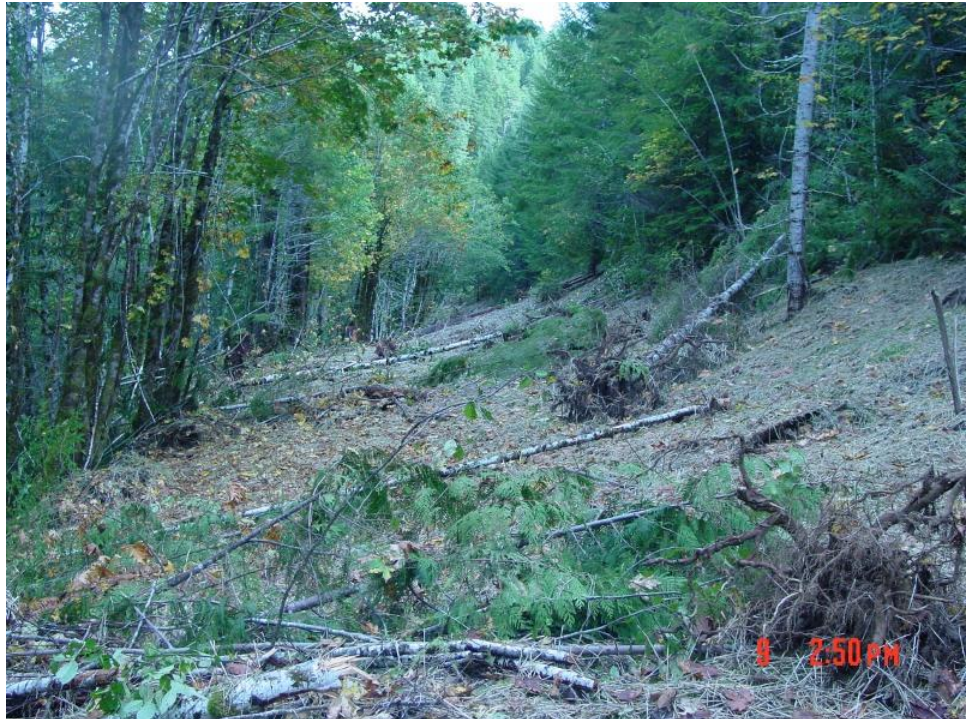
Figure 13. A decommissioned road in the Olympic National Forest. This road has been recontoured.
