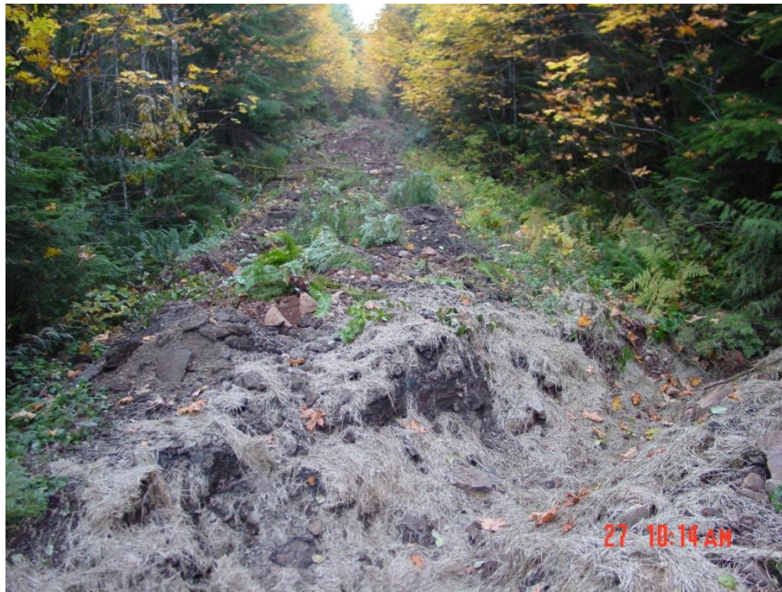
Photo C. Tilled road with water bar.
