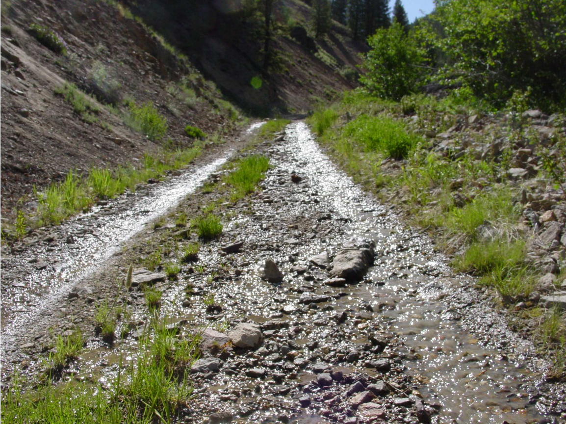
Photo 1. View looking east up the road adjacent to Coon Creek at a location approximately 500m from Monumental Creek. Notice the steep hillside on the left, and the berm on the right. The stream bed is on the right side of the berm. Water is running down tire tracks in the road.
