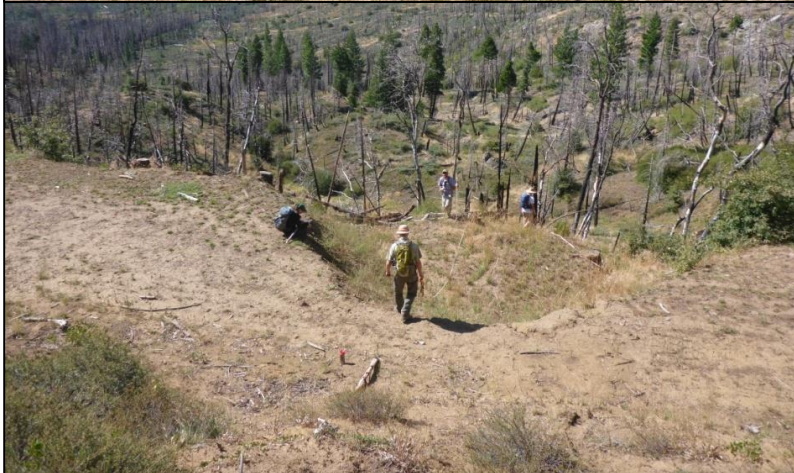
Figure 22. Fillslope failure type landslides.
