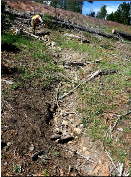
Figure 29. Gully below the outlet of a ditch relief culvert.
