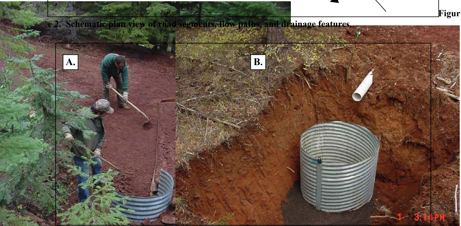
Figure 3. Photos of (A) waterbar and “ditch dam” at the downslope end of plot directing water into pipe that drains to (B) stilling pond.
