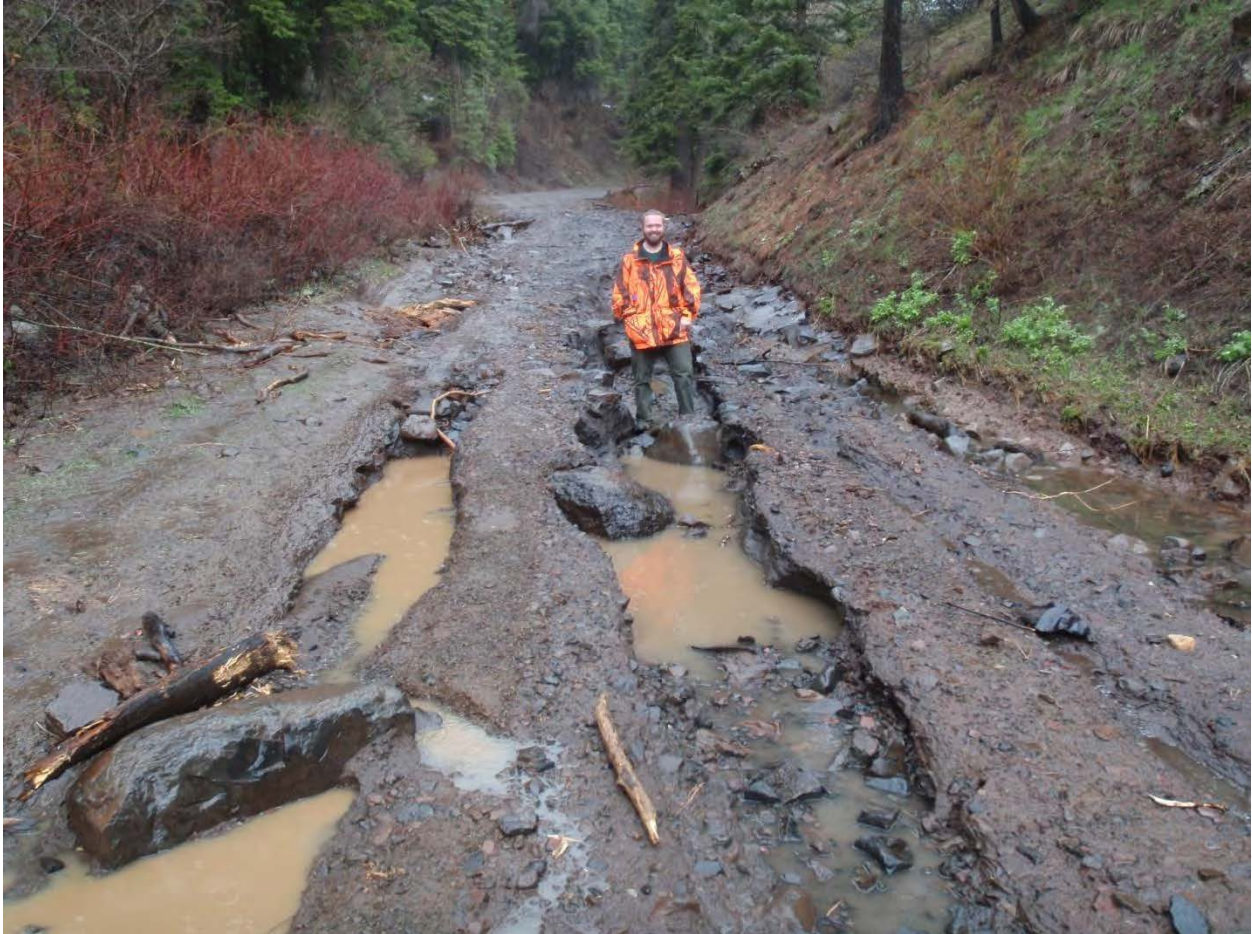
Figure 3: Damage from the April storms. The author is standing in a gullied wheeltrack where flood water was diverted down the road from the stream crossing behind the author's head.
