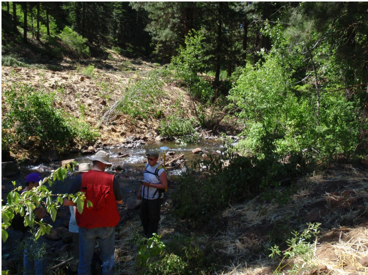
Figure 10. Example of an excavated stream crossing.
