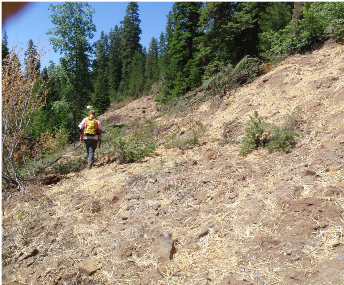
Figure 4. Photo of a typical rocky, fully recontoured road with straw mulch.
