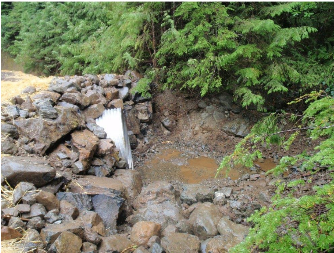
Figure 13. Stream crossing with large clast rip rap preventing the stream from diverting down the ditch.
