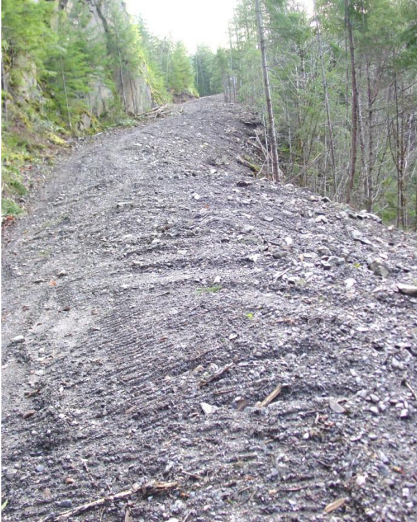
Figure 10. Insloping on Rd 2650, at the location shown in Figure 9, above.
