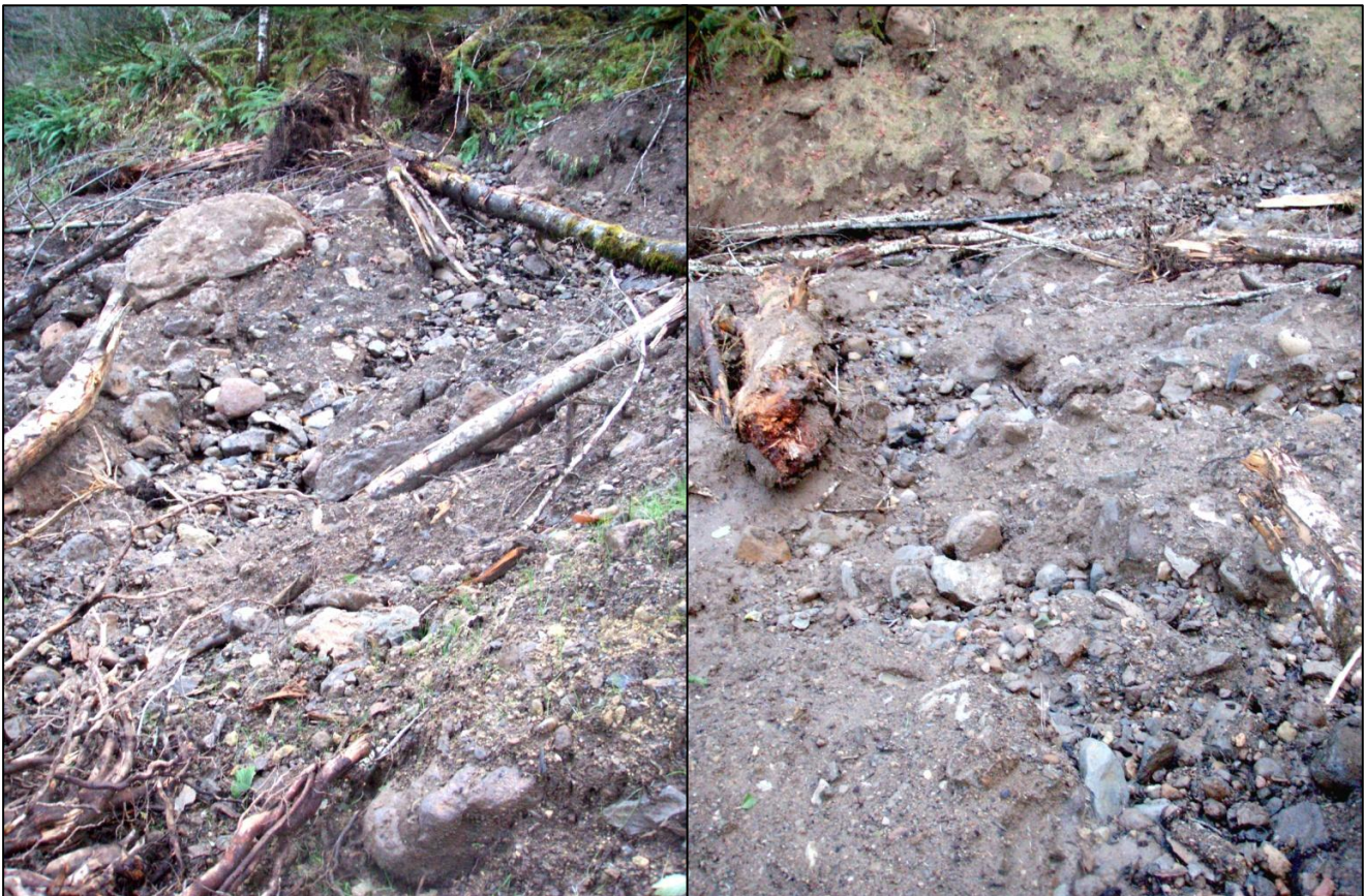
Figure 17. Spring that emits from a fill pile on NFSR 1211000. Upper part of pile (left), and channel from pile into the stream crossing (right).
