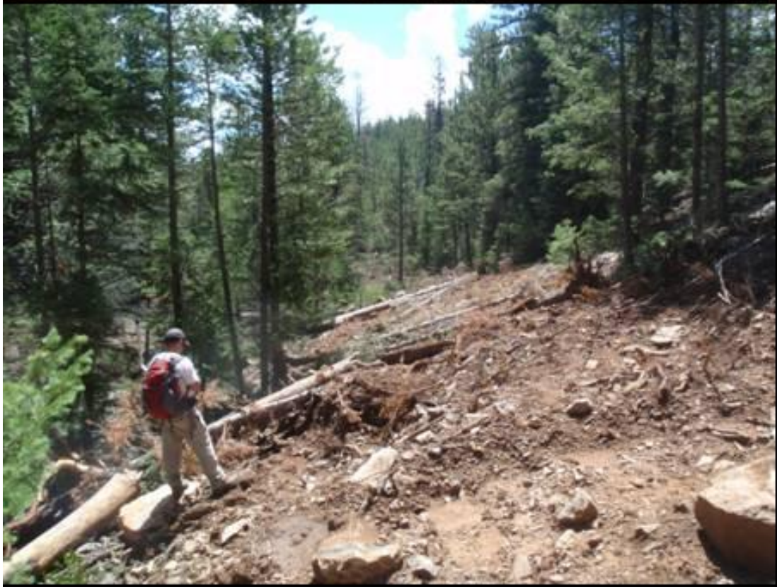
Figure 11: Typical post-storm road conditions. Tilled road on top; recontoured road on bottom.
