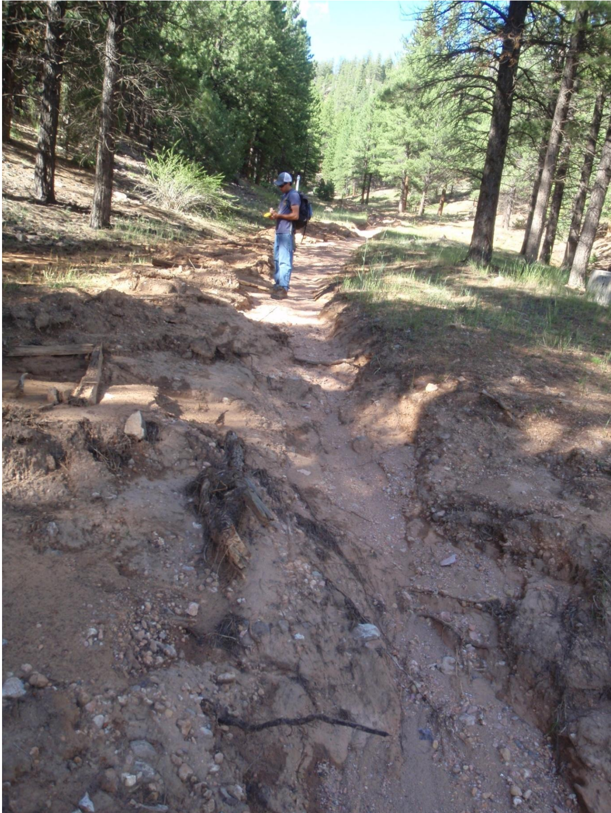
Figure 4: Storm damage on tilled road surface. The road intercepted flow in an intermittent stream channel.
