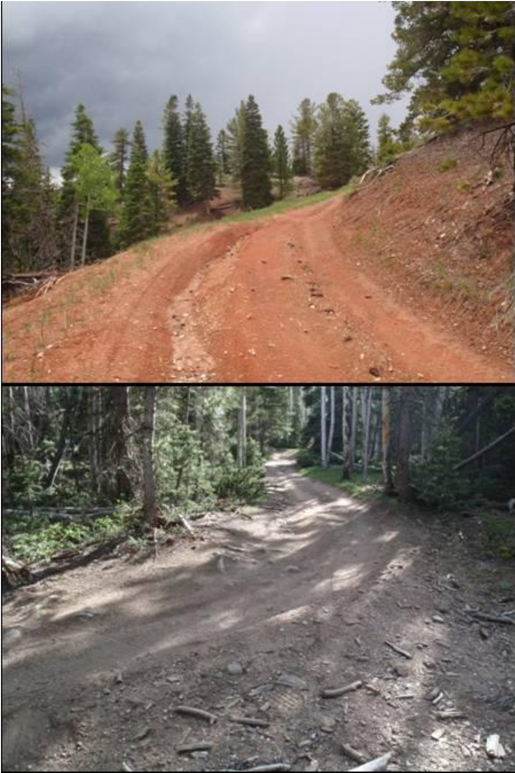
Figure 15: Typical control road sections, pre-storm.
