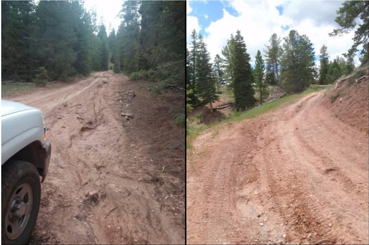
Figure 17: Typical control road conditions, post-storm.
