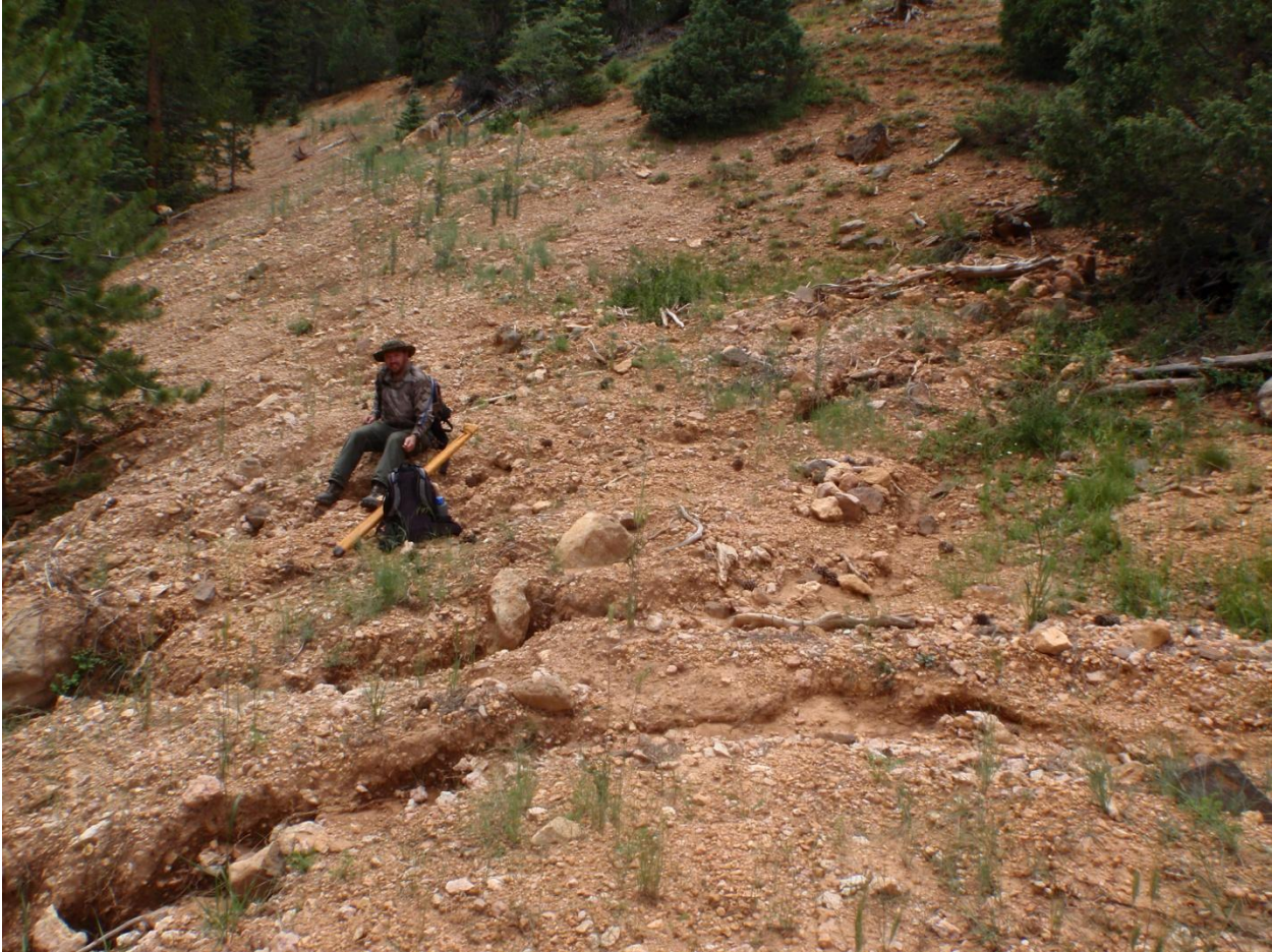
Figure 8: Gullies crossing recontoured road.
