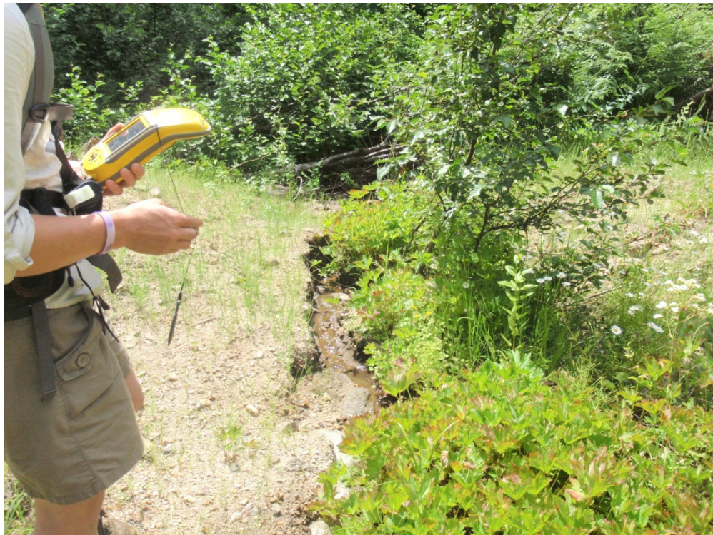
Figure 11. Fill erosion at a waterbar on road 5105 (Yakus). The erosion here is caused by the interception of discontinuous runoff and groundwater.
