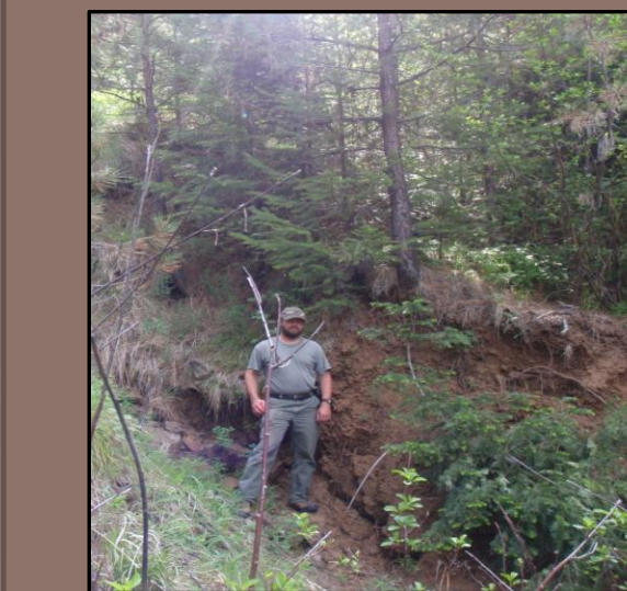
Road initiated gully
