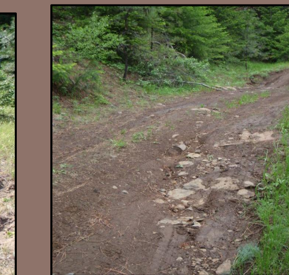
Diverted stream on road
