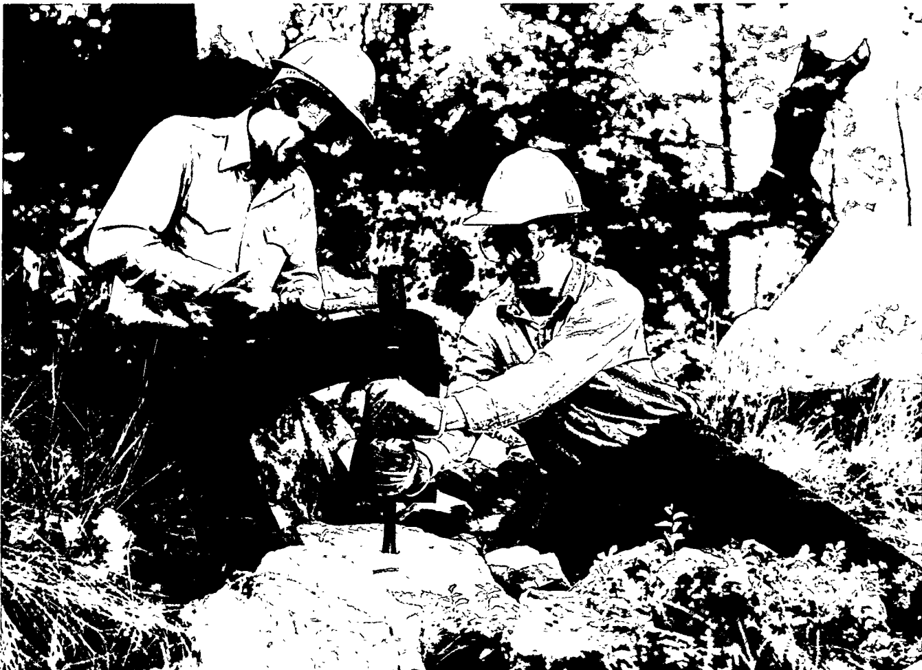
Hand drilling is an effective method for maintaining forest trails.
