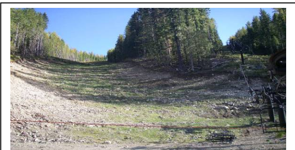
Fig. 64. 2010-excavated run after lift construction
