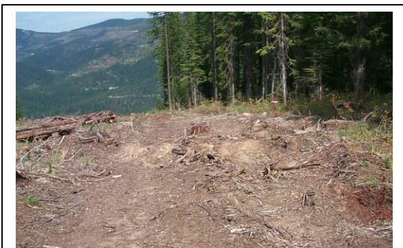
Fig. 53. 2006-waterbarred skid trail
