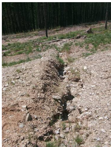
Fig. 28. 2006-eroding steep waterbar
