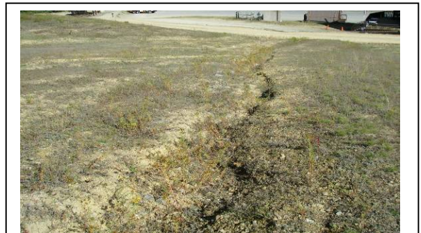
Fig. 46. 2010-erosion above Lodge
