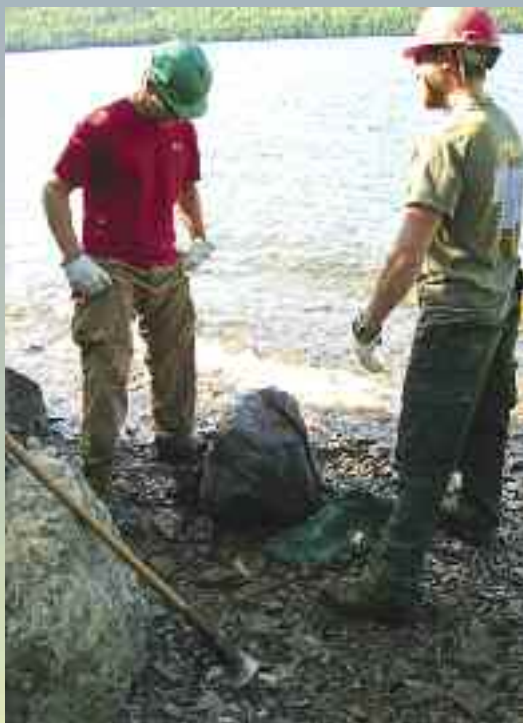
Crews conducting rehabilitation work.
