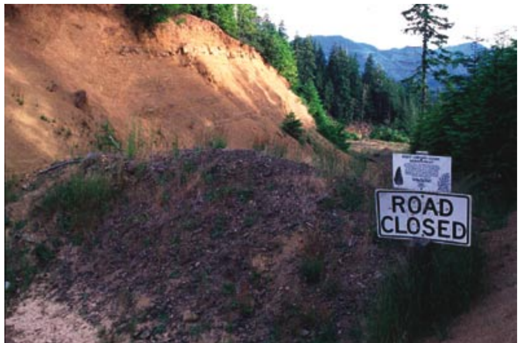
Figure 10.4—Road closed to prevent the spread of Phytophthora lateralis (permanent closure)
