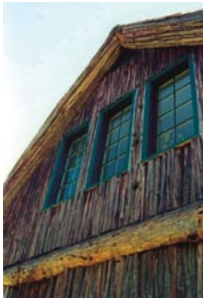
Figure 7.6—A cabin built of Port-Orford-cedar near Powers, Oregon
