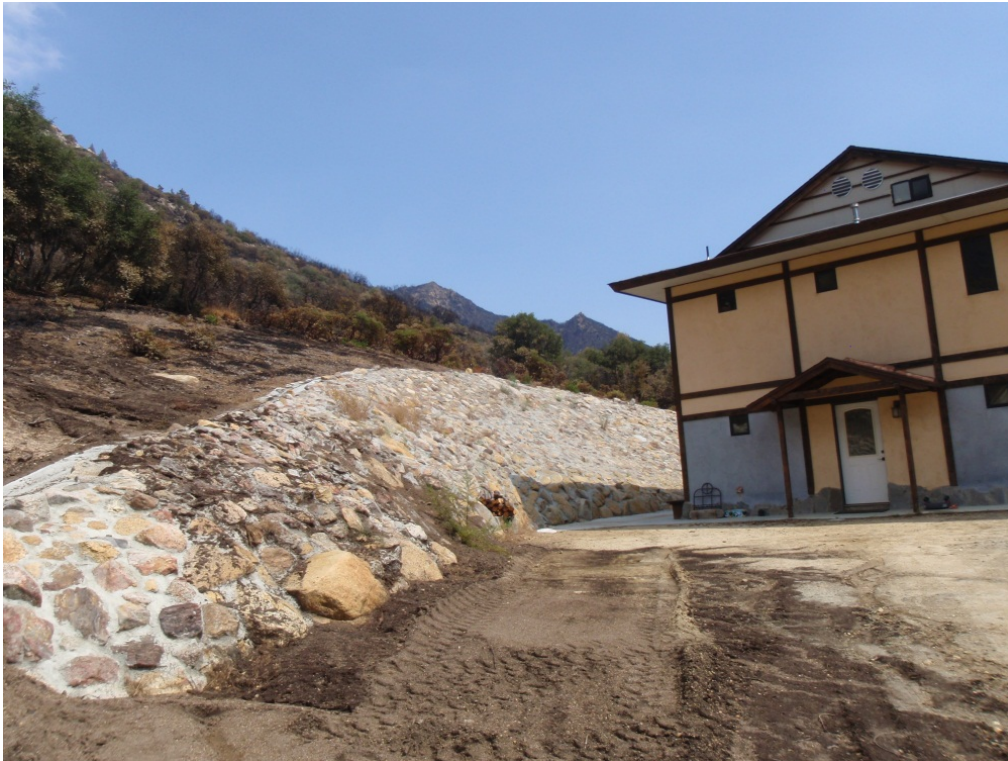
Figure 3. Fuel clearing and a home ignition zone consisting of incombustible material helped the Zen Mountain Center survive the Mountain fire. Note on left side, the fire edge came near the rock wall.
