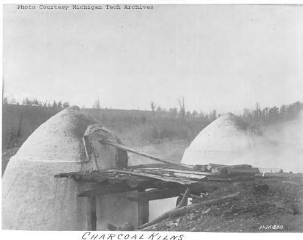
Most Charcoal Kilns were built on slopes so they would be easier to load from the top. Whitewash and mortar were used to help seal air leaks. (Photo from Keewenaw Area)
