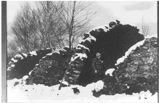
Rock Kilns, 1954. Large portions of these walls have now fallen and some kiln ruins are barely visible. Photo courtesy Braamse Family
