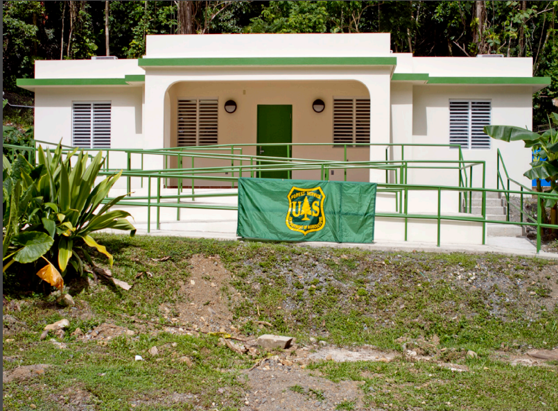
Sabana Field Research Station dormitory building. Photo credit: J.L. Hernández.
