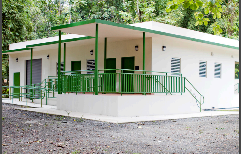
Sabana Field Research Station multi-purpose building. Photo credit: Juan Luis Hernández.
